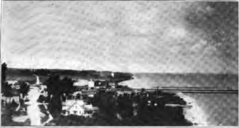
Fig. 1. View northward at Kewaunee, showing the accumulation of shore drift on the south side of the pier.
