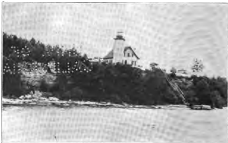
Fig. 2. Lighthouse at Eagle Point, on a rock terrace.
