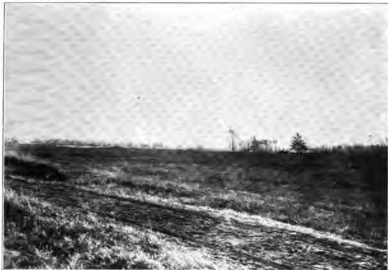
Fig. 1. Algonquin beach ridge near Cormier station.
