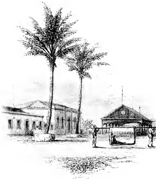
CUSTOM-HOUSE AT BENGUELA.
