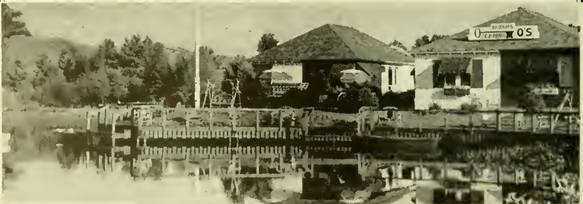
Glimpse of Keough's Cabins from the West
