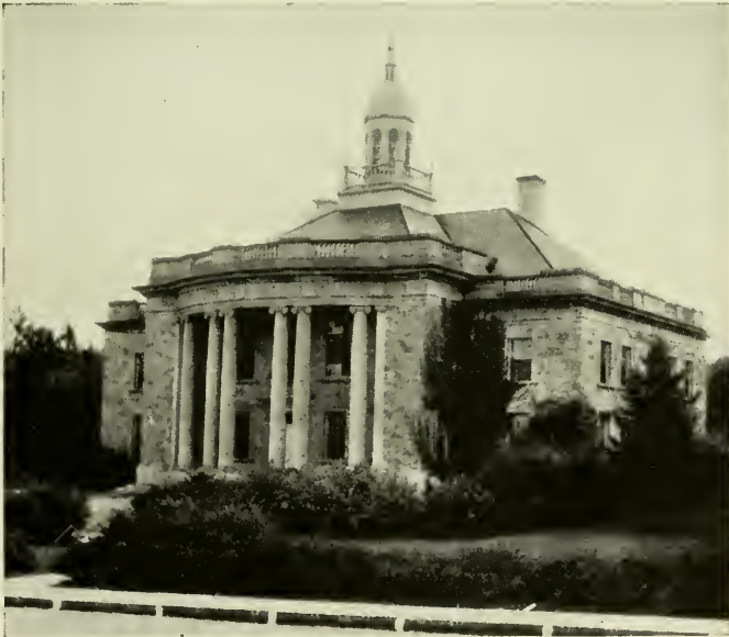
Community Building at Ticonderoga
