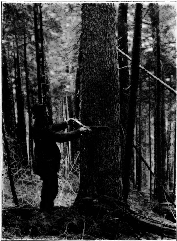
MEASURING TIMBER WITH CALLIPERS.
