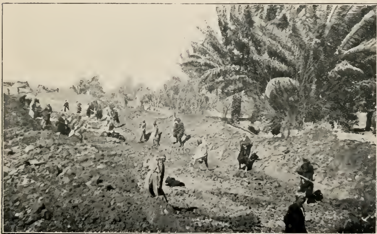
SILT CLEARANCE : ARABS AT WORK.
