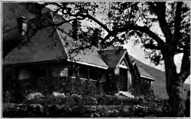
Cottage Hospital, Srinagar
