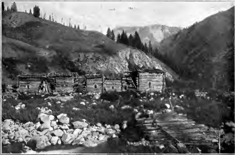
Huts and Bridge near the Zogi La
