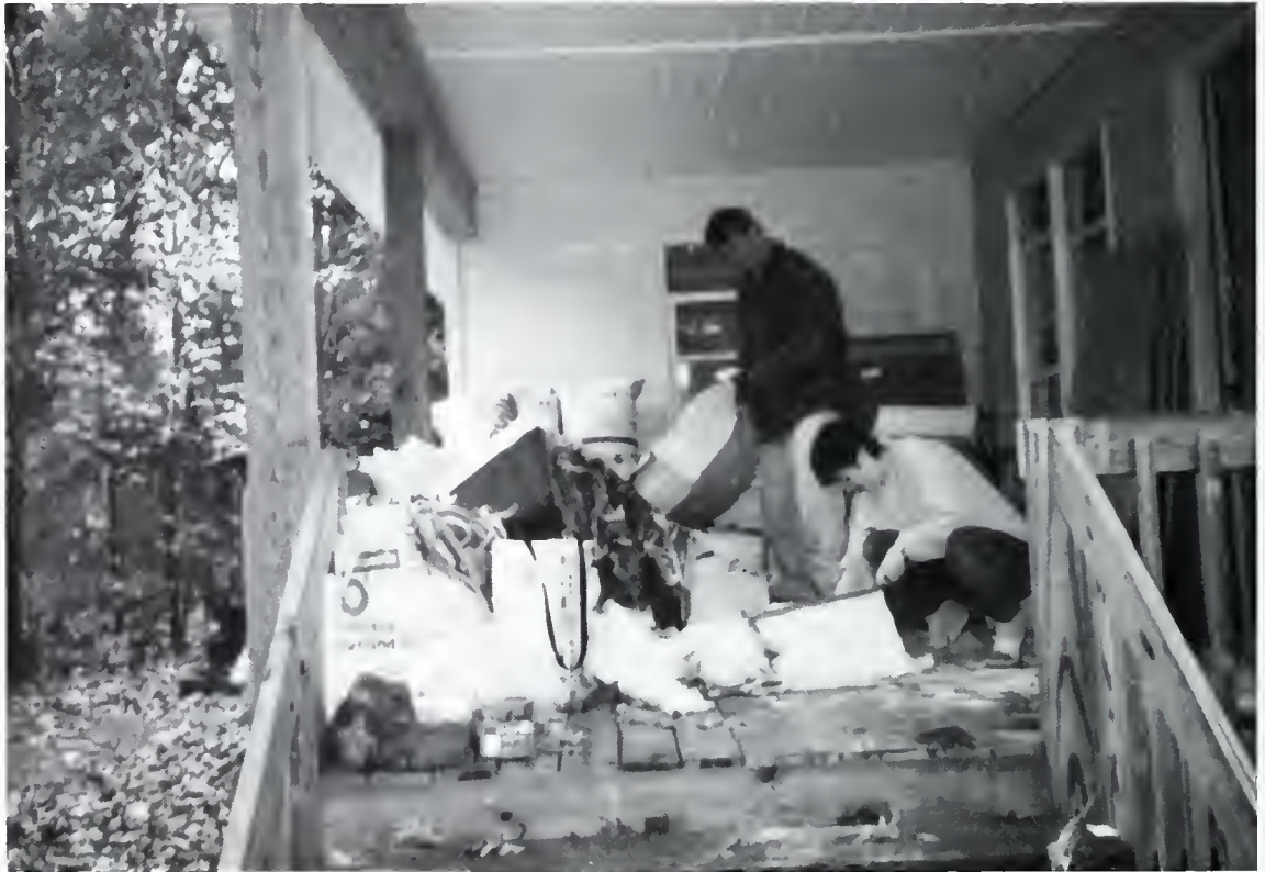
4 — Jessica & Scott working for Habitat For Humanity 5 — Eric Bush helping out
