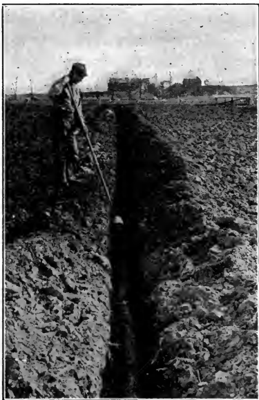
Fig. 59. Laying tile with the tile hook.
