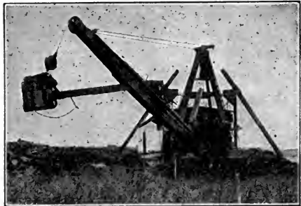
Fig. 66. A floating dredge for digging open ditches.
