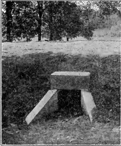
Fig. 97. Concrete culvert after the plan of Fig. 96.
