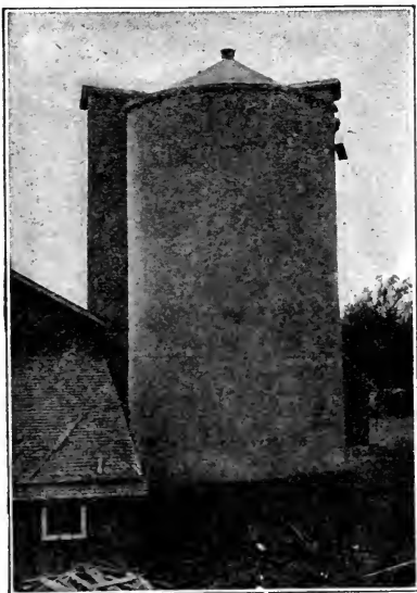
Fig. 295. A monolithic silo with concrete roof.
