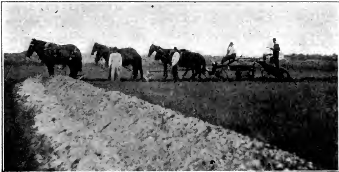
Fig. 62. Filling the ditch with a road grader.
