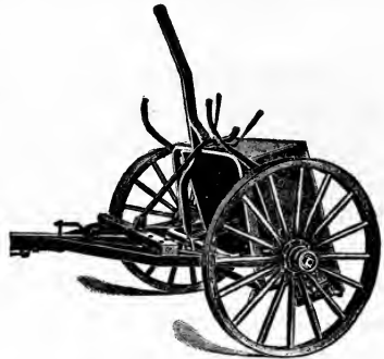
Fig. 90. Wheel scraper, dumped.
