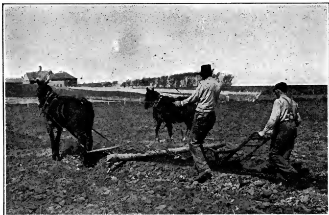
Fig. 61. Filling the ditch with a plow.
