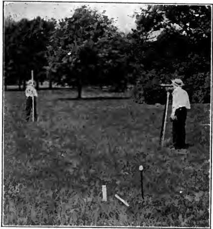
Fig. 50. Taking levels in making a survey.
