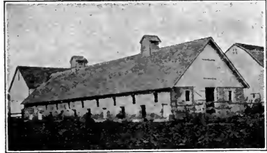
Fig. 270. A gable-roof hog house made of concrete blocks.
