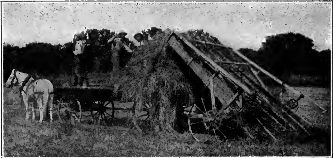
Fig. 167. A fork hay loader at work.
