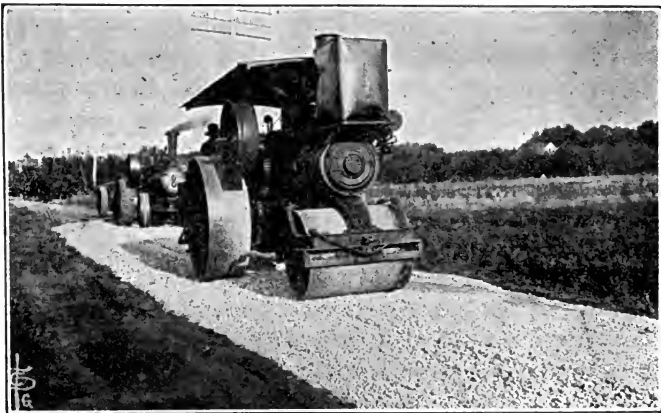
Fig. 84. Rolling the first course of stone.
