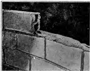
Fig. 297. The wall of the Iowa silo.
