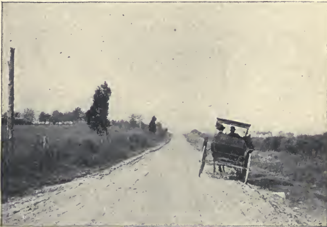
The same road improved.
