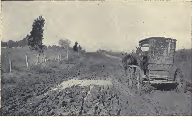
An earth road that needs improving.
