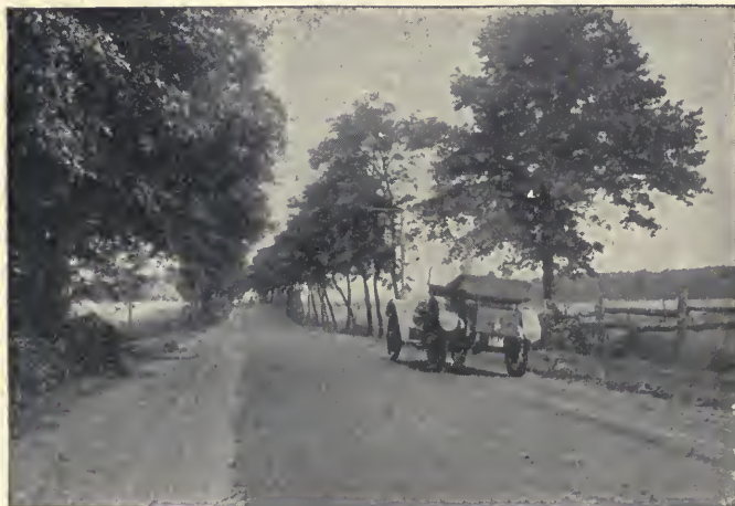
Bituminous macadam road in New Jersey.
