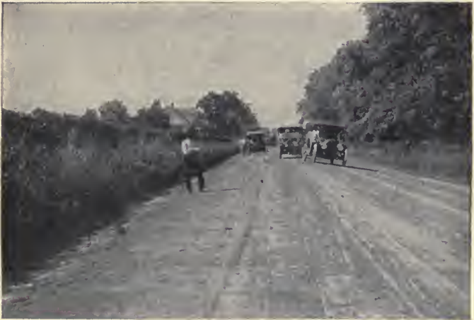
Earth road in Kansas.
