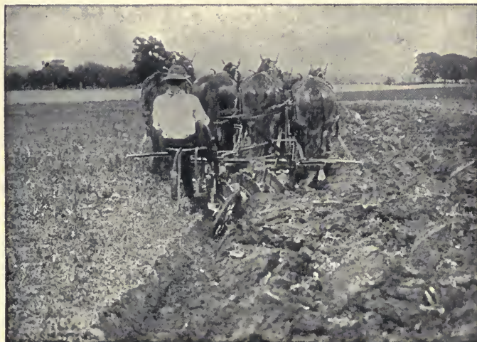
A deep tilling plow, with two disks.
