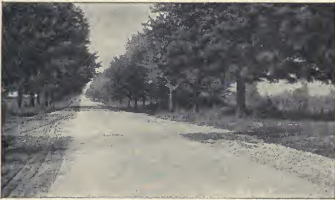
Concrete road near Detroit.
