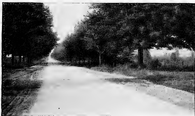
Concrete road near Detroit.
