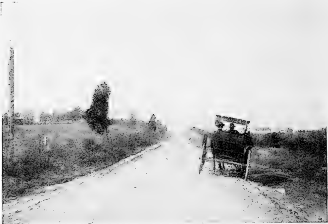
The same road improved.
