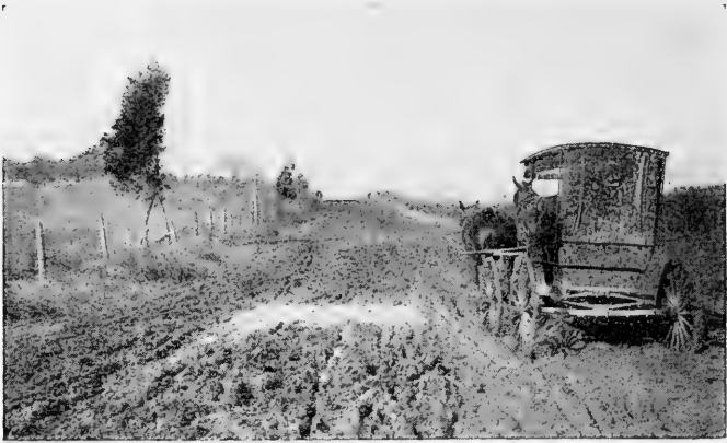
An earth road that needs improving.
