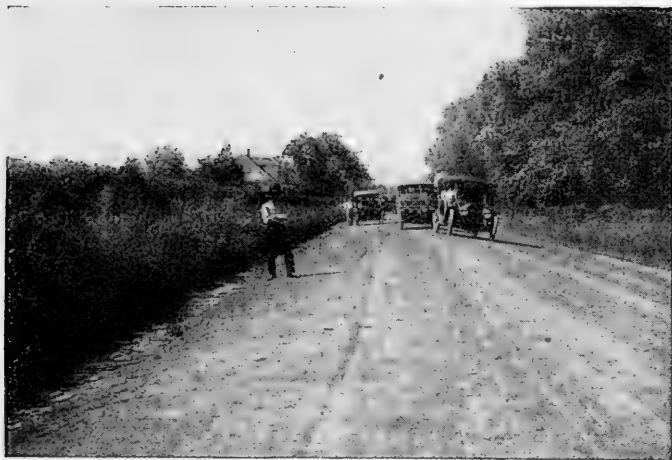
Earth road in Kansas.
