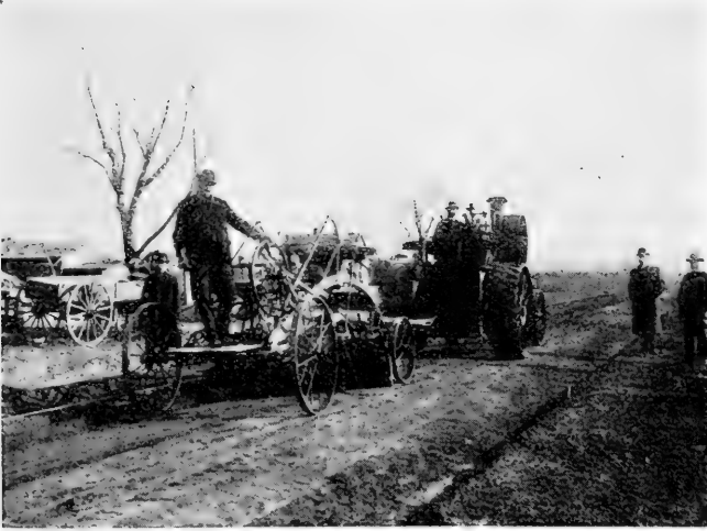
Preparing foundation for macadam road.
