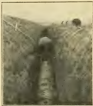
Placing the tile in trenches.
