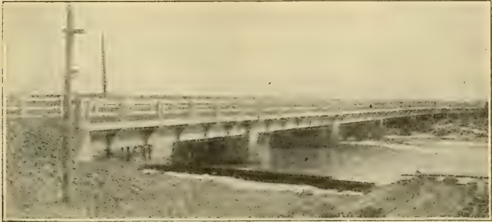
A concrete bridge. The permanency of this structure is plainly evident.
