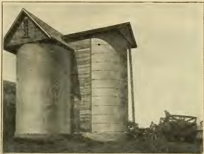
Filling a silo. A blower is used to elevate the material from the cutter to the silo.
