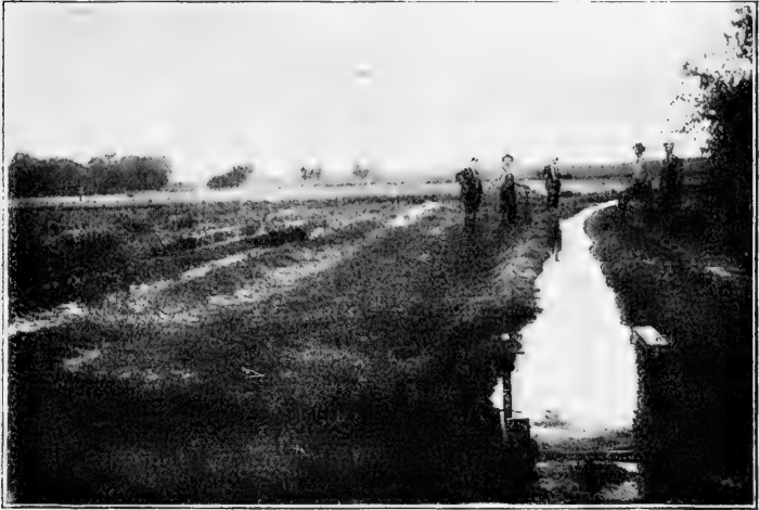
A lateral carrying water to a distant part of the field.
