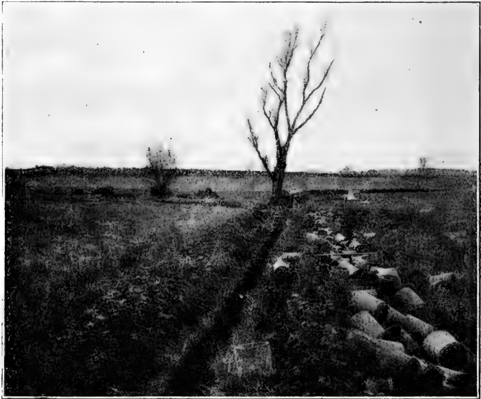
Draining a field. Notice depth and relation of ditches, and distribution of tile.
