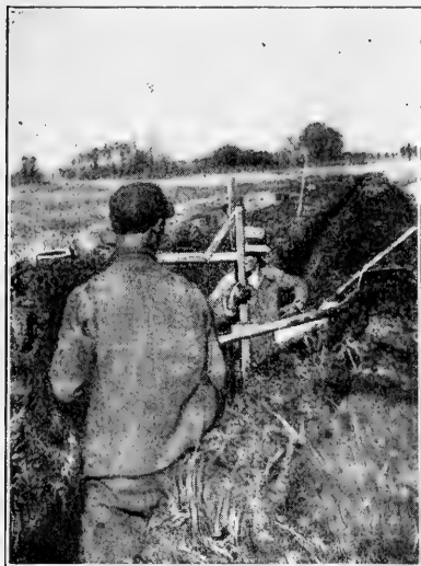
Digging a drainage ditch.
