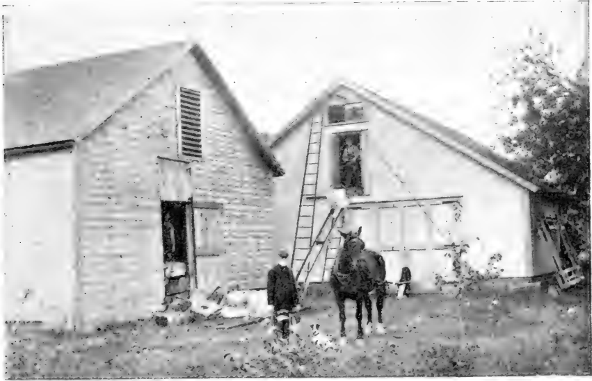
Rear of Mr. Clark's Cold Storage—Filling Ice Box.
