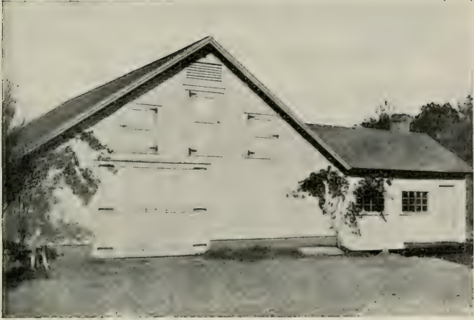
Storage house of John W. Clark, North Hadley, Mass. (front view)
