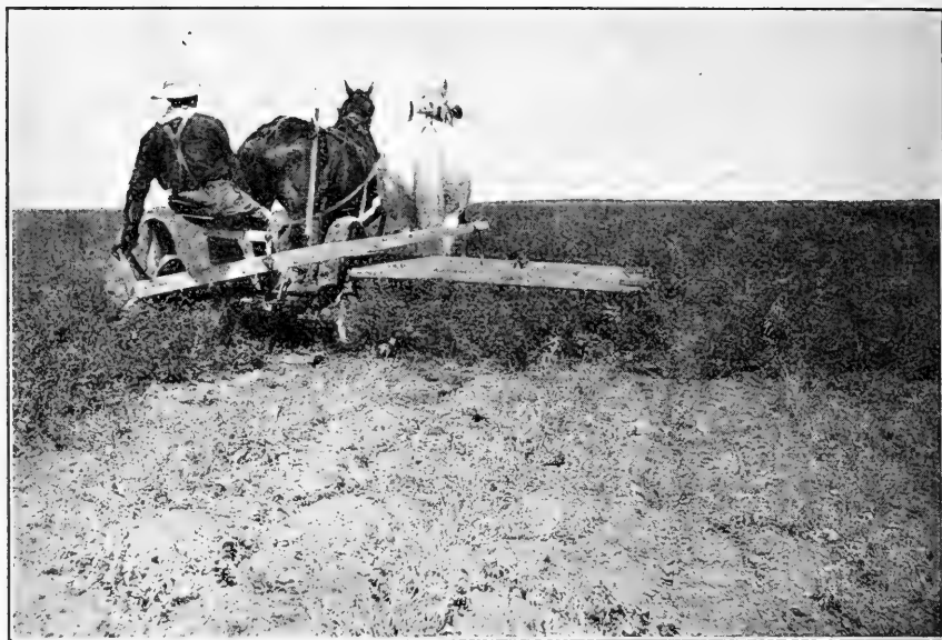
Fig. 7.—Mowing machine with dropper attachment in operation in a field of alfalfa in cultivated rows in western Nebraska. The rows in this case are one-half mile long. (Brand and Westgate—B. P. I. Circ. 24—U. S. Department Agriculture.
