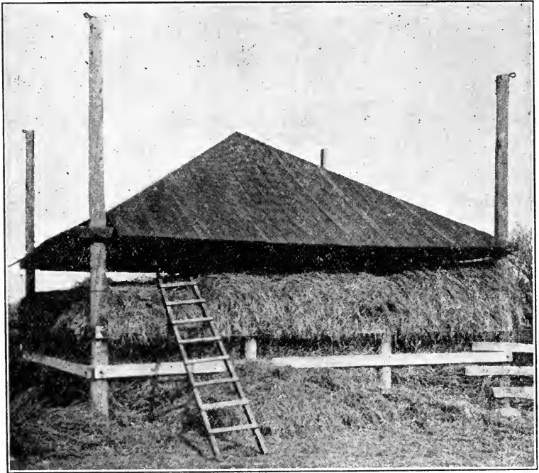
FIG. 100. A hay shed with an adjustable roof. It is about twenty-five feet square, the corner posts are smooth and strong, and it is well bolted together. The roof is raised or lowered with rope and pulley, and is supported on iron pegs that fit in holes bored in the corner posts at regular intervals. With this arrangement the rain can not blow in on top of the hay, whether the shed be full or nearly empty. A practicable small-scale method of storage near or in the feed lots.
