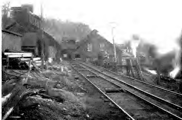
FIG. 2.—MINING PLANT AT OCEAN, NO. 1.
