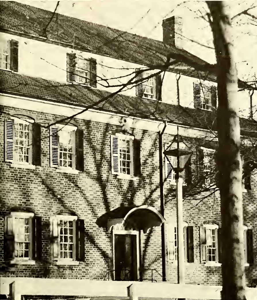
The restoration of South Hall on Church Street — Completed in 1966.
