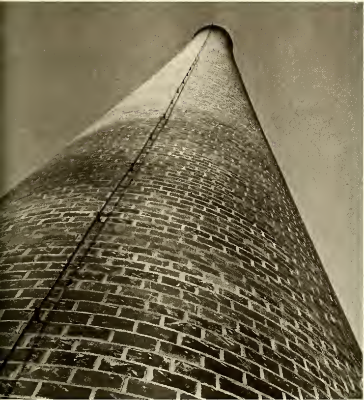
The Steam Plant, completed in 1956, enabled the construction of additional campus buildings to pro- ceed. The plant has since been converted from coal to gas.
