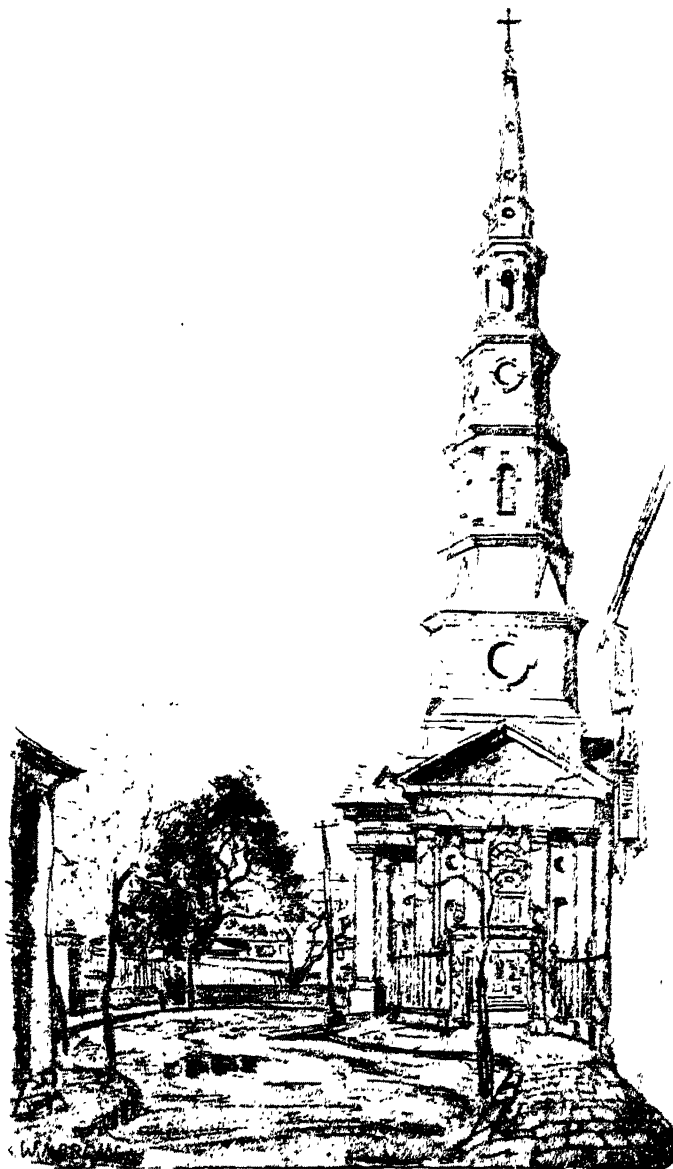
St. Philip's is the more beautiful for the open space before it, and the graceful outward bend of Church Street in deference to the projecting portico
