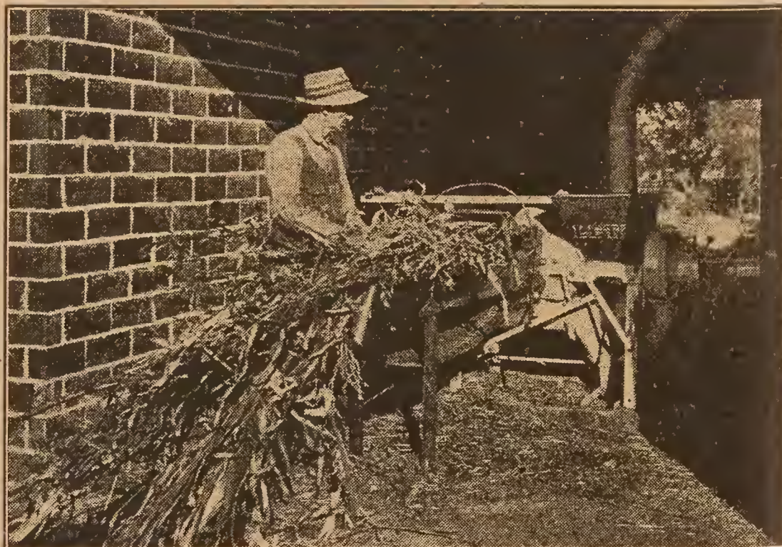
A feed grinder that will grind and mix grain and roughage.
