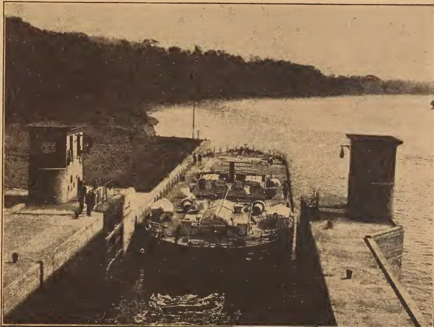
—Courtesy N. Y. S. Department of Public Works When a boat comes to a "hill" in the barge canal, it is taken into a lock, great water tight doors are closed behind it and water is pumped into the lock. When the proper level is reached the doors ahead of the boat are opened and the boat proceeds.
