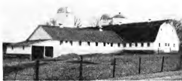
Fairlawn Farm's buildings are clean, well-built, efficient.
