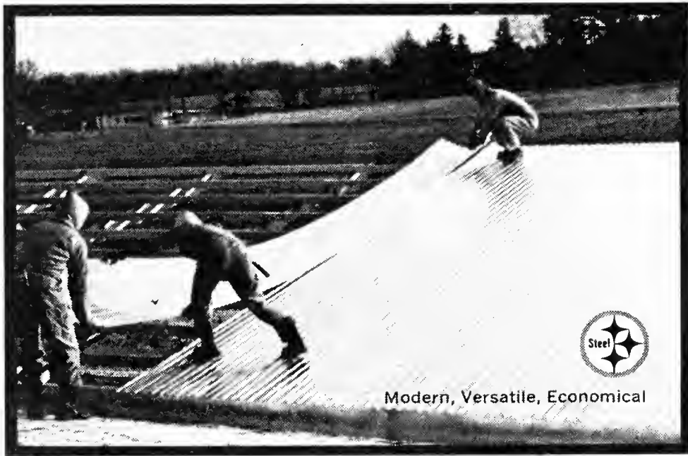
Republic Rigid-Rib Sheets shown are 28 feet long.
