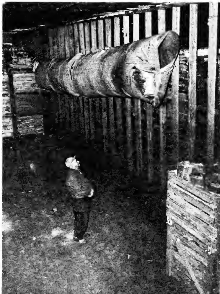
Merton Colby uses a plastic "pipe" to distribute air in his storage. Floor of storage is sand.
