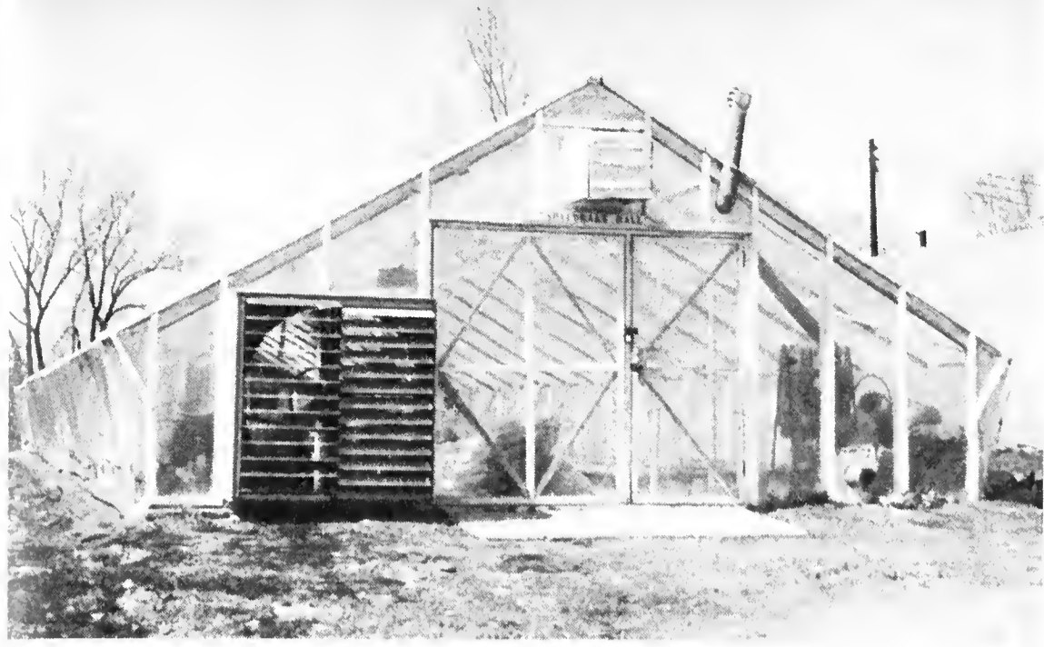
A door that is eight feet wide allows room for truck or tractor to enter. Note big ventilating fan at left.
