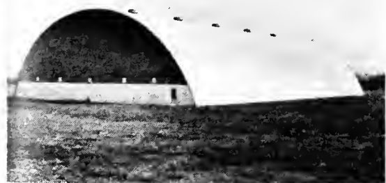
Storage on Sodoma Brothers Farm was once a theater at Sampson AFB.
