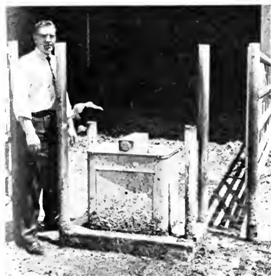
Walk-throughs 13 inches wide in the fences of the various lots at the Utah State University dairy farm, allow workers to go in and out without opening the gates. Posts of 3-inch iron pipe are set in the floor or footings of the waterer.
