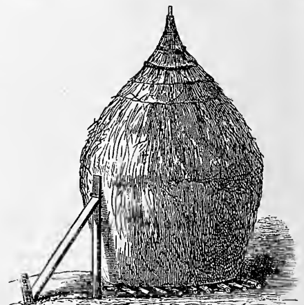
A STACK BRACED TO PREVENT LEANING.
