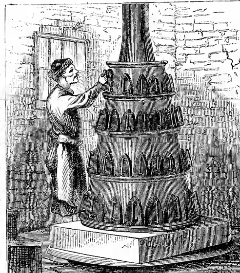
Fig. 5.—STOVE FOR HEATING IRONS.
