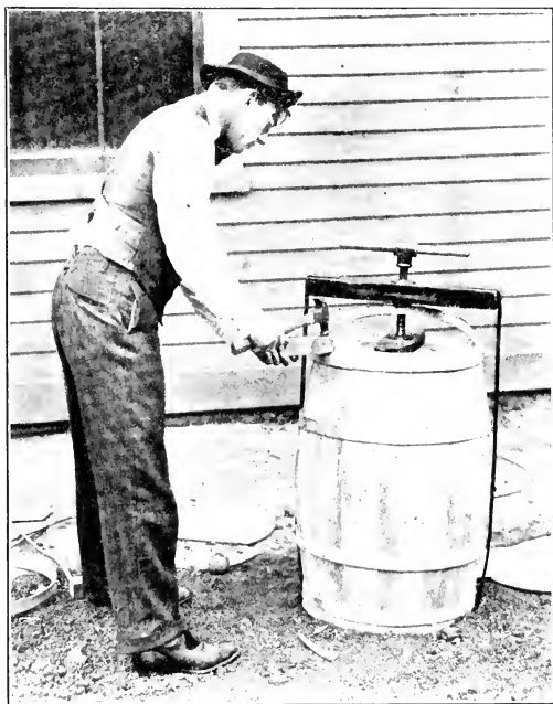
HEADING UP THE BARREL.—SCREW PRESS
