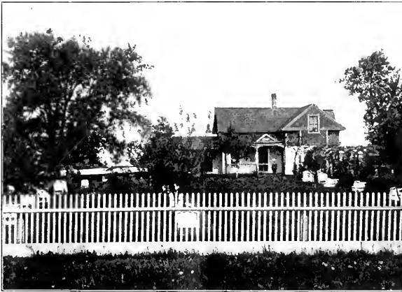
APIARY AND RESIDENCE OF W. E. BAKER, LIVINGSTON CO., ILL. (See next page.)
