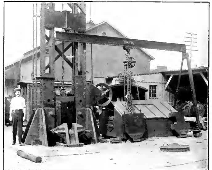
New Drop Testing Machine; Baltimore & Ohio.
