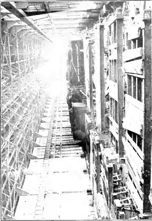
General View of the Tank Shop: Beech Grove Shops.
