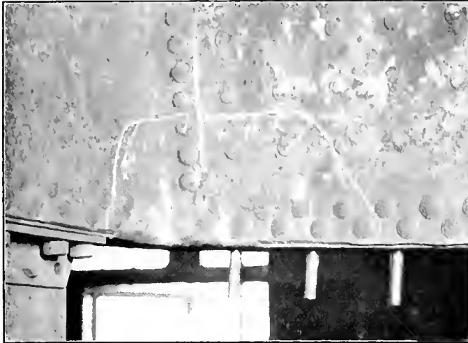
Fig. 7—Defective Firebox Sheets Repaired by Electric Welding.
