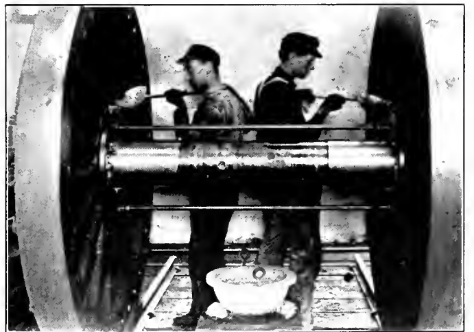
Fig. 11—Pouring Babbitt Hub Liners.
