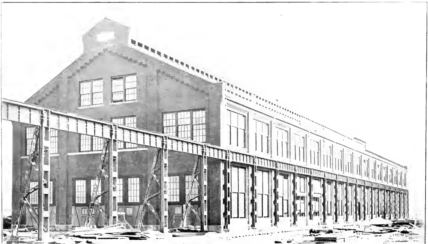
General View of Planing Mill and Cabinet Shop.
