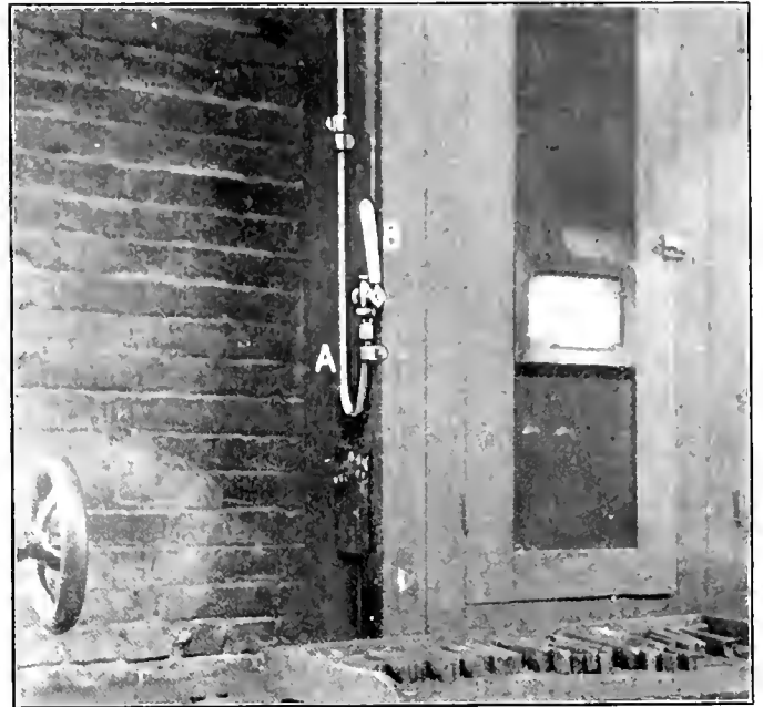
Fig. 6—One of the Air Valves in the Shop for Stopping the Engine in an Emergency.
