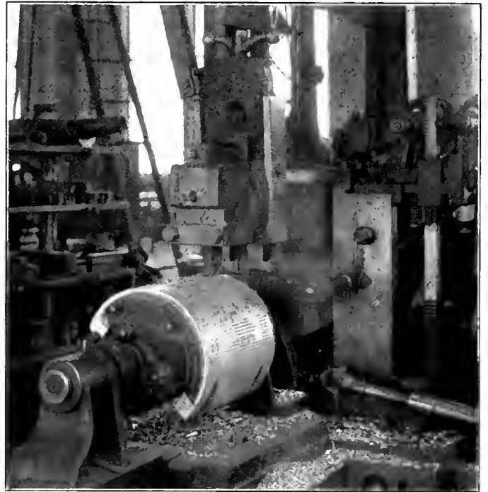
Fig. 3—Finishing a Crown Brass on a Draw Cut Shaper.
