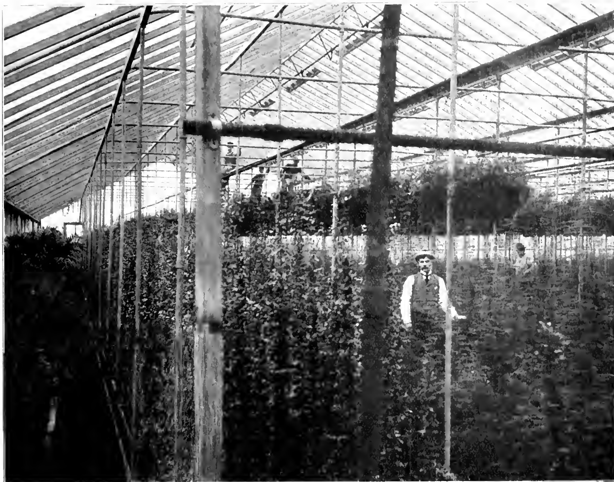
VIEW IN THE RANGE OF ASPARAGUS HOUSES OF ALBERT F. AMLING, AT MAYWOOD, ILL.
