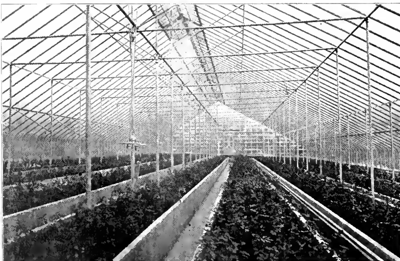
INTERIOR OF NEW PIERSON-SEFTON HOUSE, AT BRIARCLIFF.
