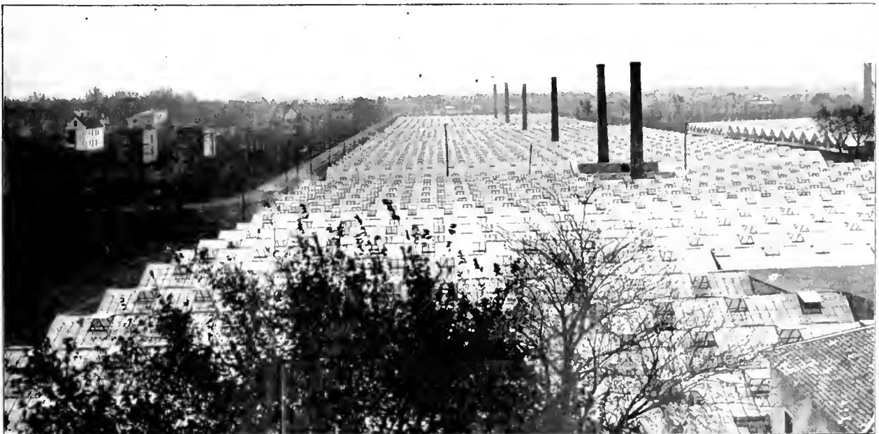
THIS VIEW SHOWS ONLY A PART OF OUR RANGE OF 1,000,000 FEET OF GLASS.
