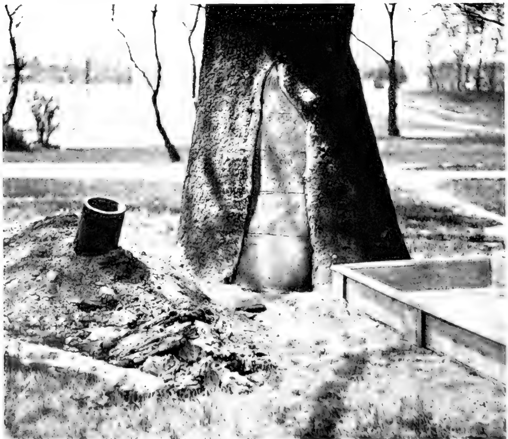
THE JOB WELL DONE WITH THREE WAGON LOADS OF CONCRETE AND CEMENT TO FILL THE HOLLOW.
