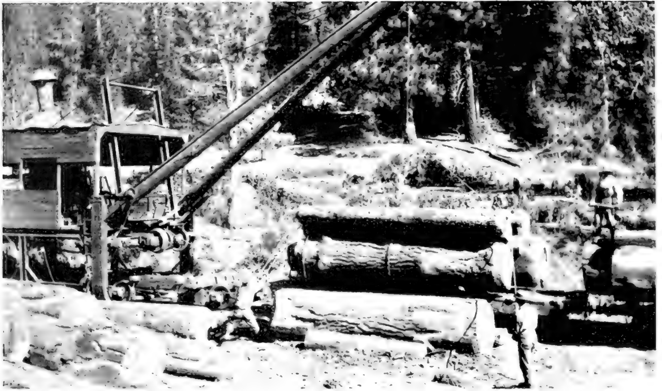
STEAM LOADER ON MARCH LUMBER COMPANY'S LOGGING RAILROAD, PLUMAS NATIONAL FOREST.
