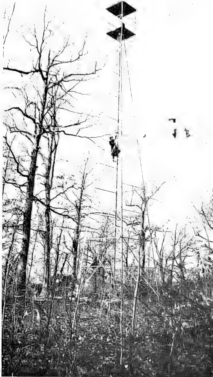
SHOWS LOOKOUT TOWER ON McGOWAN'S POINT. THESE PICTURES SHOW THE NEED OF A HIGH TOWER ON THE OZARK NATIONAL FOREST, BECAUSE OF THE HIGH TREES SURROUNDING. THESE TREES THAT ARE NEAR WILL BE FELLED TO PREVENT DAMAGE BY REASON OF THEIR FALLING AGAINST IT IN A HEAVY WIND STORM. McGOWAN'S POINT, ARKANSAS.
