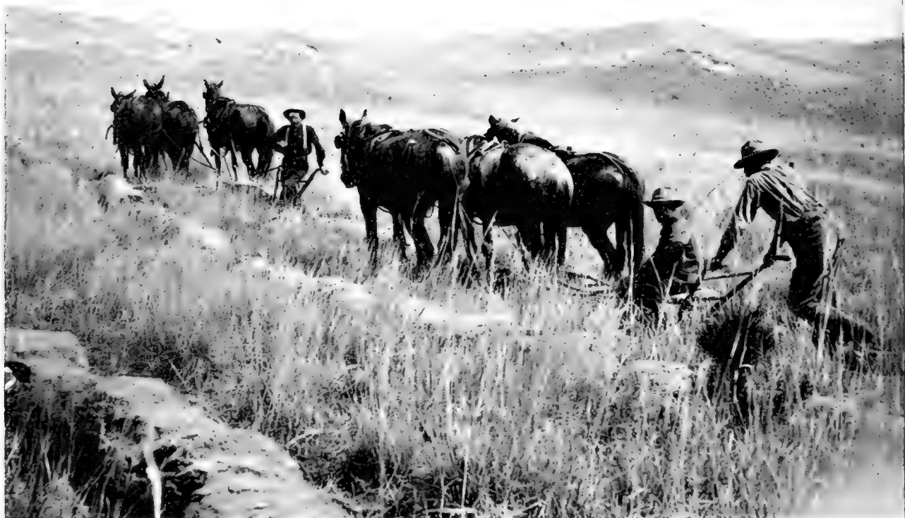
THE PLOW WITH TRENCHER FOLLOWING
