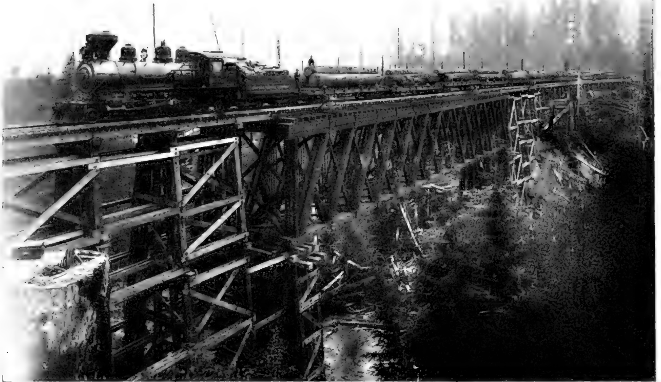
BRIDGE OVER WEST FORK OF TATSOP RIVER, 130 FEET ABOVE THE RIVER. WITHIN ONE MILE ON THIS SAME ROAD IS THE TWIN OF THE BRIDGE. IT IS ESTIMATED THAT THE LAST 1\frac{1}{2} MILES OF THIS ROAD, INCLUDING THESE BRIDGES, COST NEARLY $100,000 TO PUT INTO OPERATION. IT IS STRICTLY A LOGGING ROAD. SIMPSON LOGGING CO., SHELTON, WASH.
