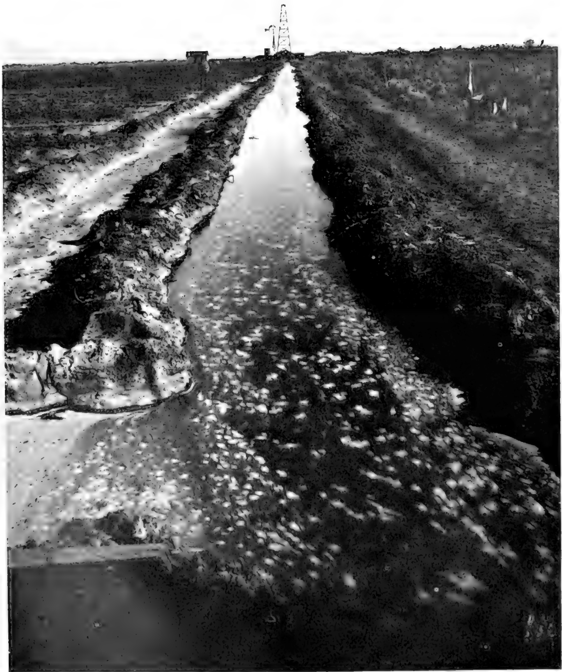
IRRIGATION DITCH SUPPLIED BY WELL, PUMPING 1,300 GALLONS OF WATER PER MINUTE NEAR DEMING, N. M.
