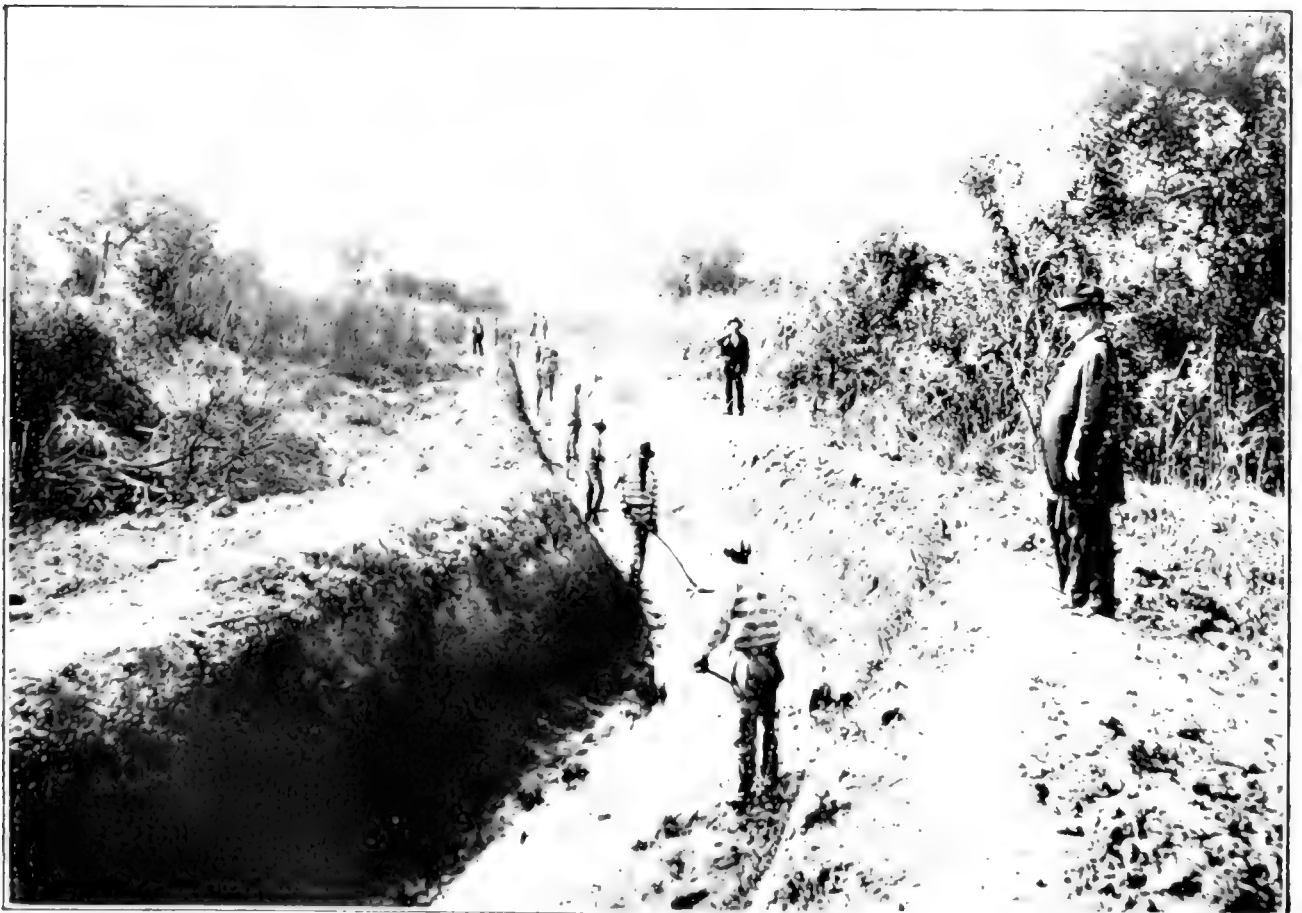
CONVICTS WORKING IN DRAINAGE DITCH, HOLBECK'S SWAMP, NEAR CHARLESTON, S. C.
