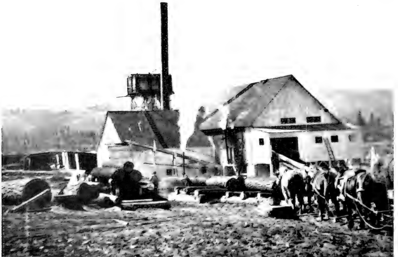
FEATHER RIVER LUMBER CO. MILL NO. 2 OPERATING ON GOVERNMENT TIMBER ON THE PLUMAS NATIONAL FOREST. CUT 40,000 PER DAY.
