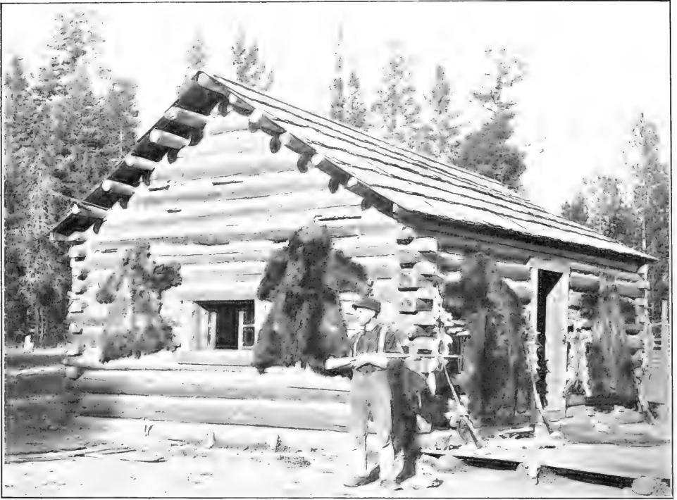
FOREST SERVICE RANGER STATION.
