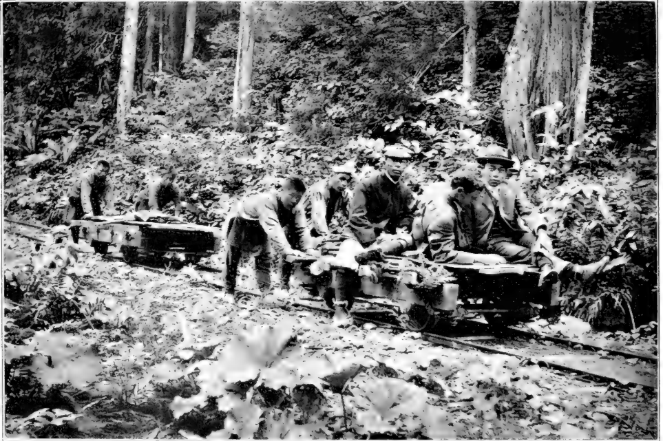
A LOGGING RAILROAD THESE CARS ON THE ODATE GOVERNMENT FOREST ARE RUN MAINLY BY GRAVITY
