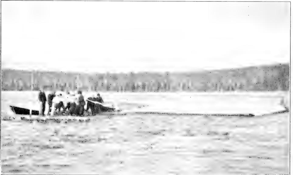
WINDING IN A BOOM BY HAND
