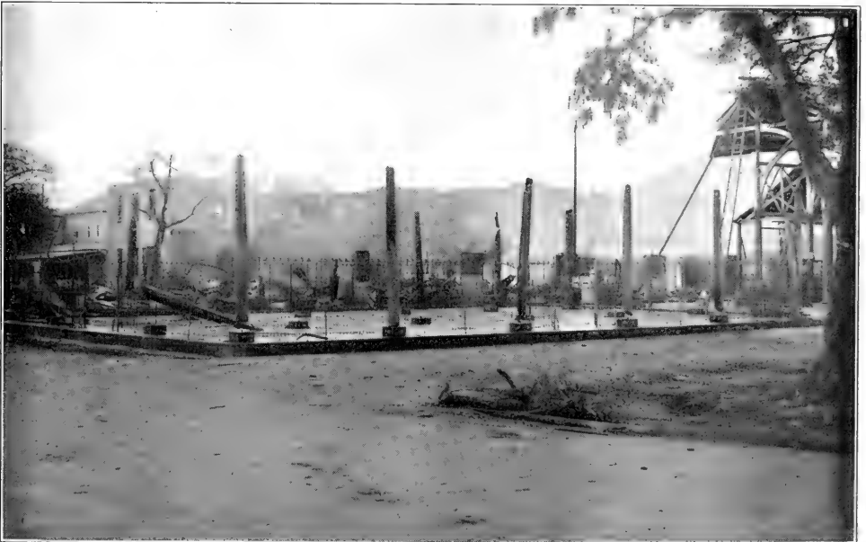
THE PUBLIC MARKET BURNED. THE SHELLS OF THE GERMAN CRUISERS SET FIRE TO THIS MARKET AND IT WAS BURNED TO ITS CONCRETE FOUNDATIONS.
