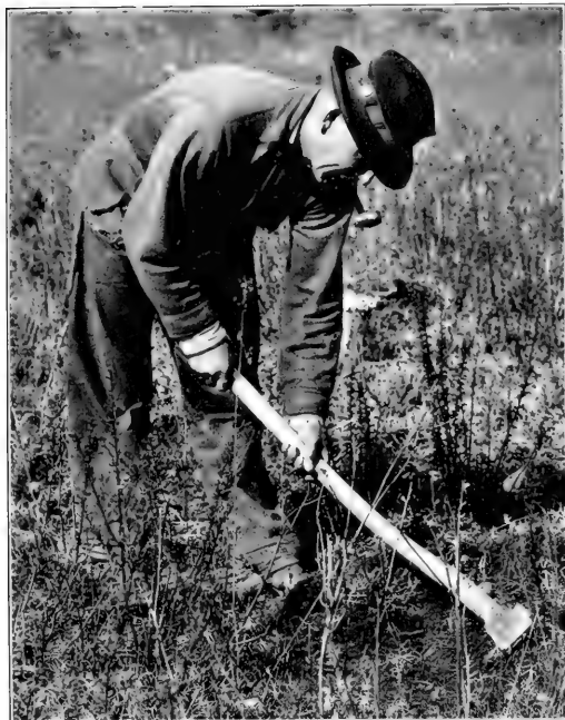
REMOVING TURF AND DIGGING HOLE
