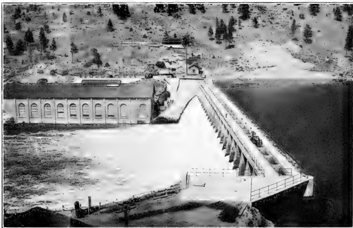
HAUSER LAKE PLANT OF THE MONTANA POWER COMPANY
