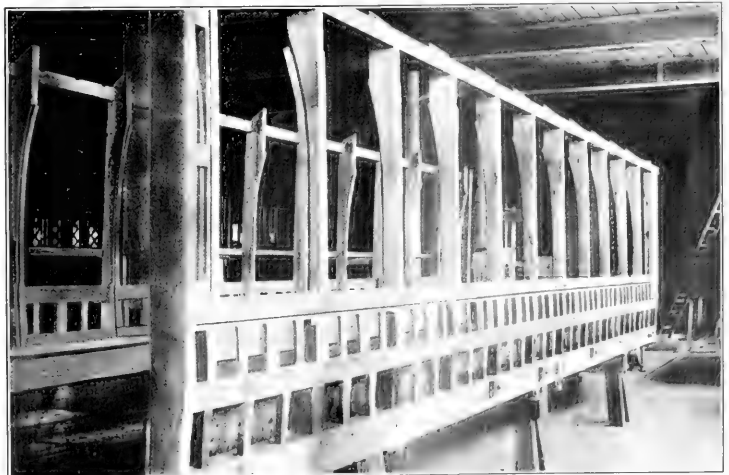
STREET CAR CONSTRUCTION
