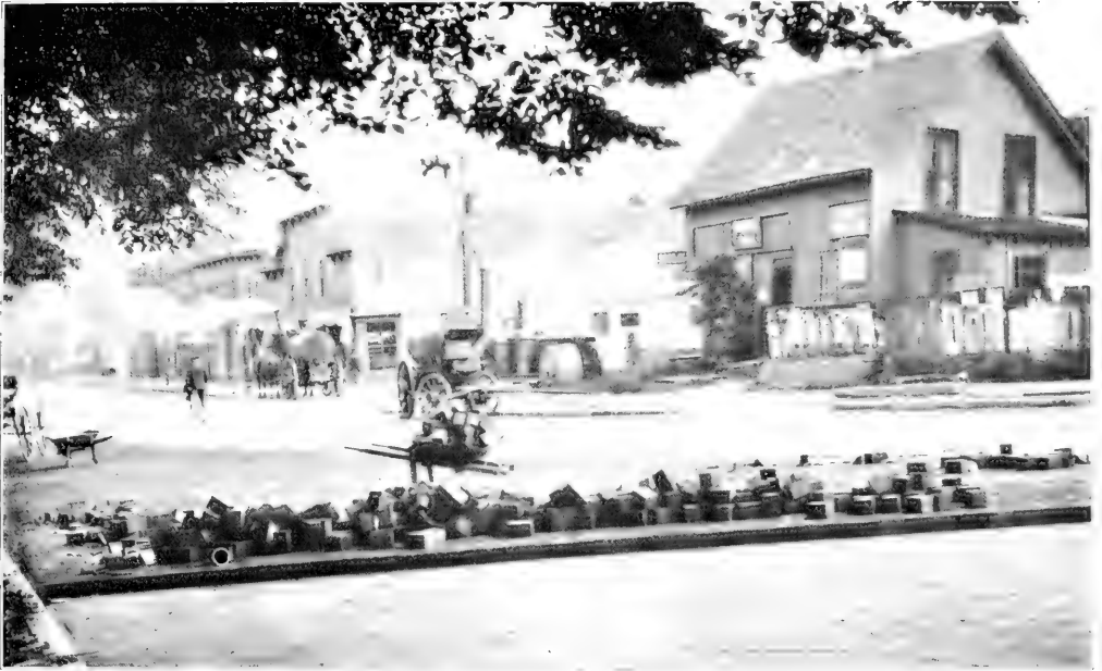
LONGLEAF PINE USED LARGELY FOR WOOD BLOCK PAVEMENT
