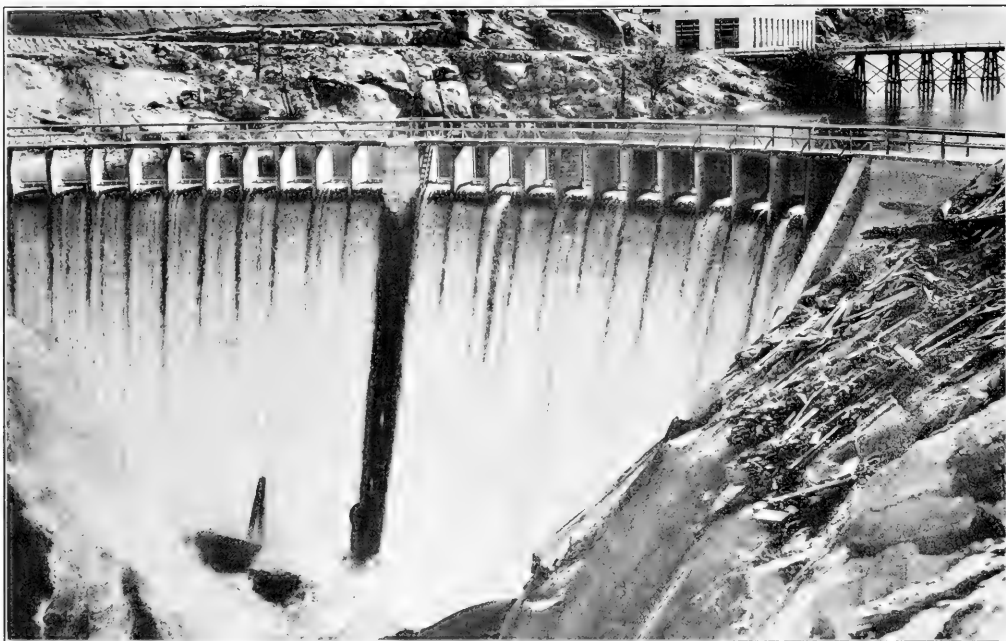
DIVERSION DAM FOR PLANT NO. 2 OF THE PACIFIC LIGHT AND POWER CORPORATION
