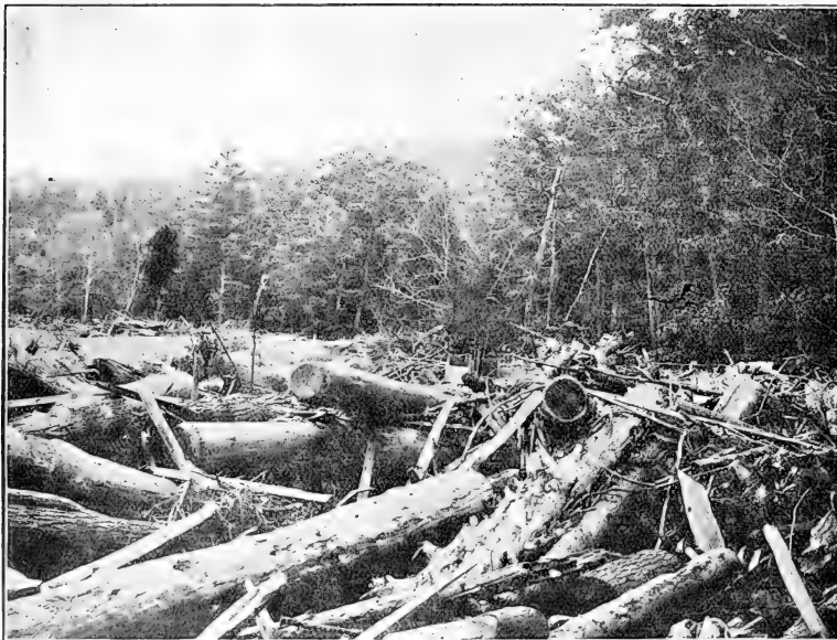
Debris from Wreck of Sawmill and Log Boom on Linville River, by Floods, in Western North Carolina, in Region of Proposed National Forest Reserve
