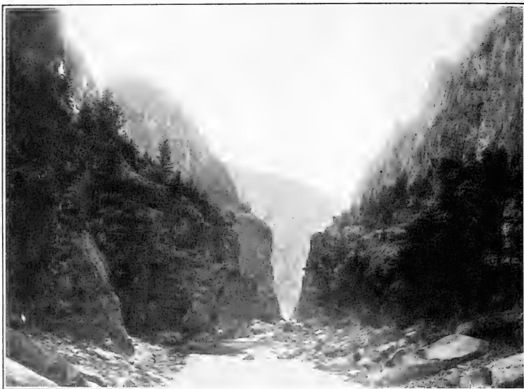
Shoshone Dam Site. Highest dam in the world; to be built at this point by U. S. Reclamation Service. Dimensions: 310 feet high, 85 feet long at bottom, 200 feet at top.
