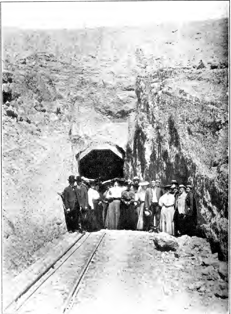
Congressional inspection party at the mouth of the Gunnison Tunnel, Colorado, now 7,000 feet within the mountain. One of the most interesting engineering projects the Reclamation Service is engaged upon.
