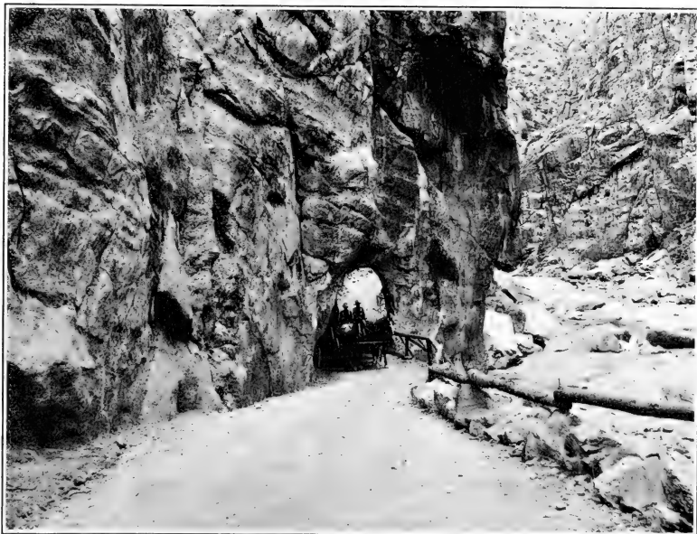
Detail View of Complete West Entrance of Tunnel just below Shoshone Dam Site on Canyon Road, Shoshone Project, Wyoming
