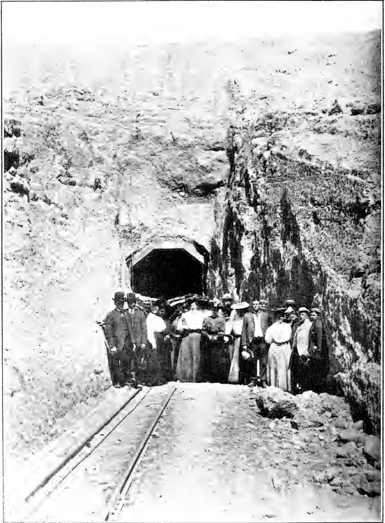
Congressional Inspection Party Mouth of Gunnison Tunnel, Now 15,000 Feet Within the Mountain.
