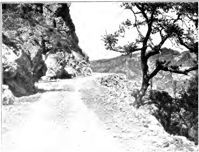
The Roosevelt Road, leading from Phoenix, Mesa and Tempe, Arizona, to the Roosevelt Dam (Salt River Project). This road is 62 miles in length, over 40 of which extend through the Canyon of the Salt River. The road was built by the U. S. Reclamation Service and the three towns mentioned contributed $75,000 of its cost. A remarkable feature of its construction was the fact that the day labor was performed by Apache Indians, remnants of the mighty Geronimo's former band; a tremendous step in civilization this marks in turning these Indians from terrorizing the country to actually assisting in its development.
