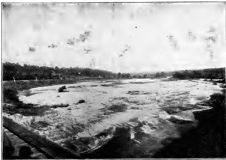
Soil Removed and White Sand Spread Over the Surface of the Catawba River Lowlands. The damages along this river from the floods of May and August, 1901, aggregated about $1,500,000.
