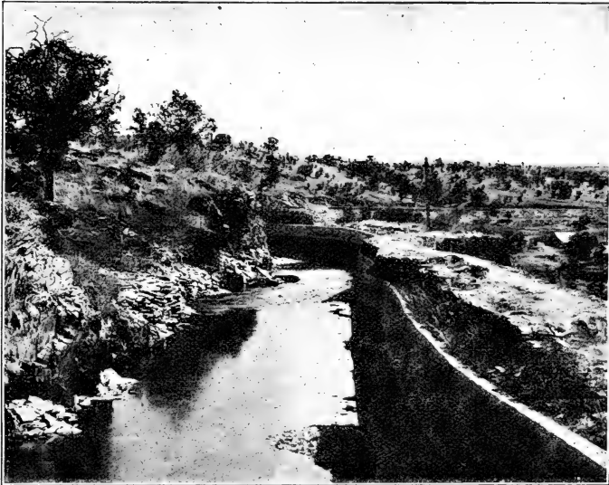
Sidehill Construction on the Bear River Canal, Utah.
