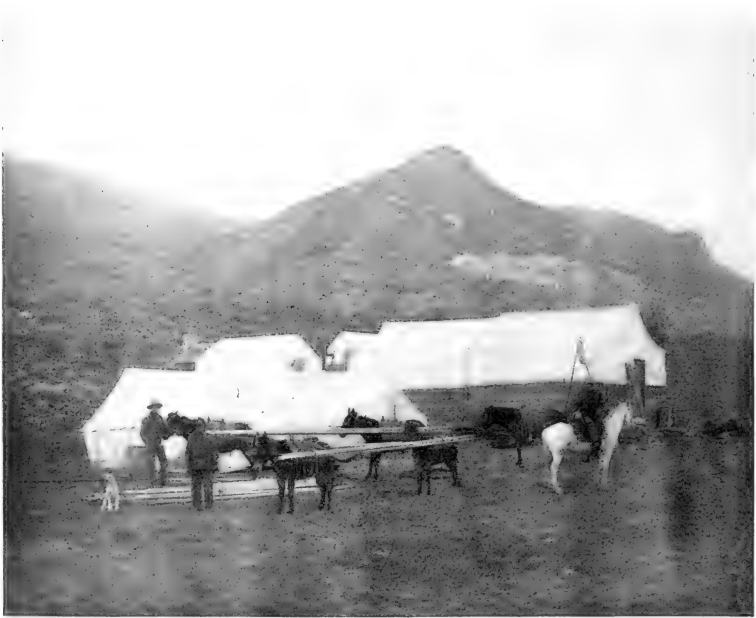
Carrying Supplies into Roosevelt, Arizona, before the wagon road was completed.
