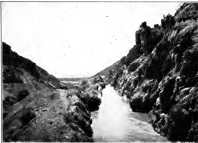
Section of Turlock Canal, California.
