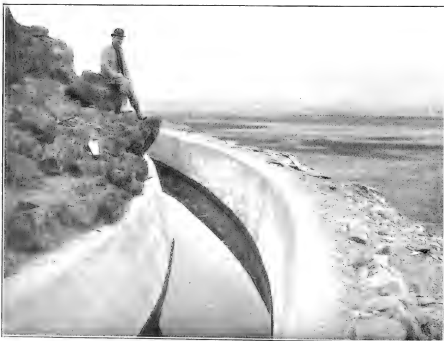
Okanogan Project, Washington. Completed Portion of Concrete Lined Canal, Showing Lands on Pogue Flat to Be Irrigated under Canal
