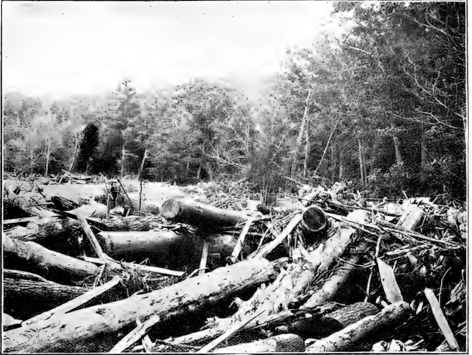
Debris from Wreck of Sawmill and Log Boom on Linville River, by Floods, in Western North Carolina, in Region of Proposed National Forest Reserve
