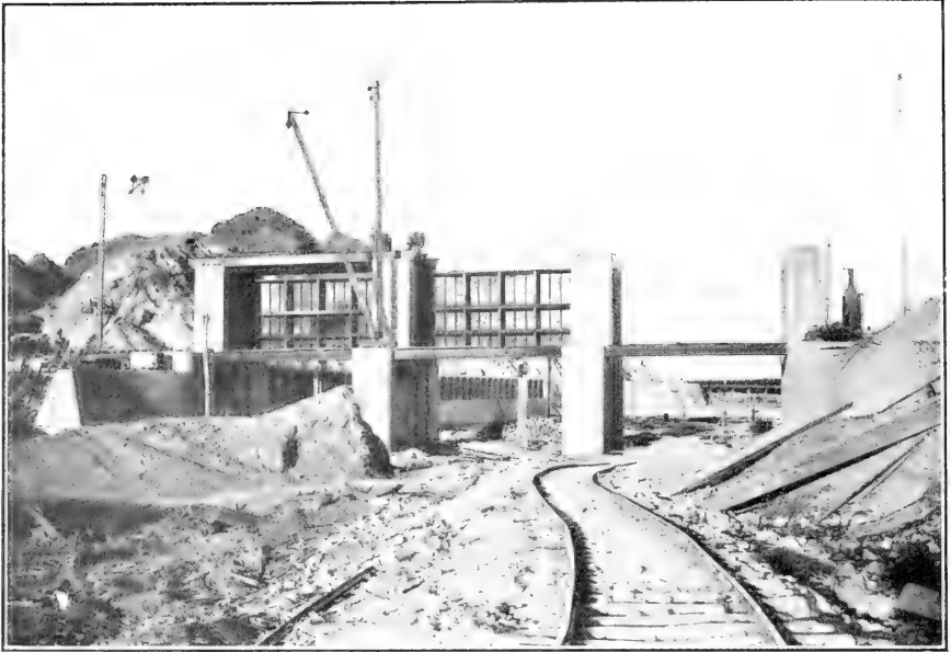
Yuma Project, Arizona. Sluiceways on California Side, 35 by 18 Feet Each. Sluiceways 200 Feet Wide on Bottom, Largest in World
