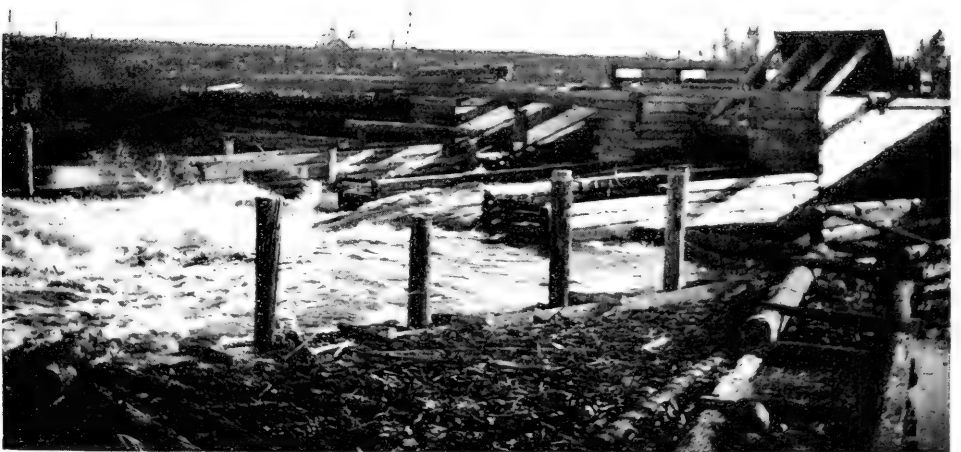
Sluiceways of a Splash-dam (Minnesota)
