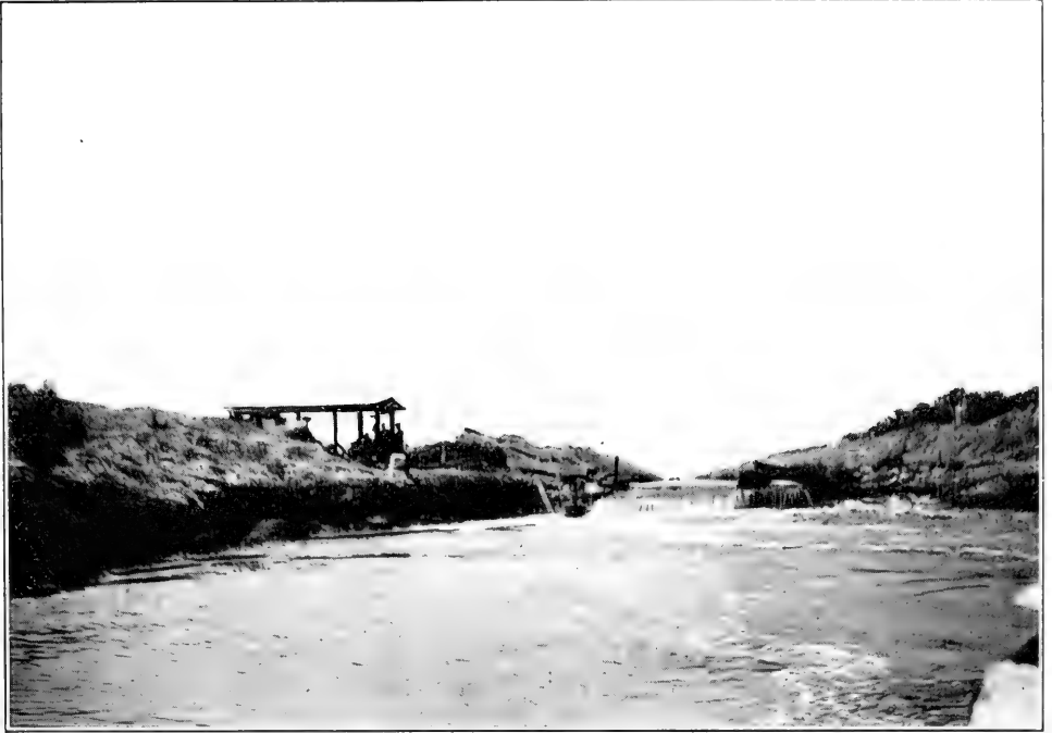
Canal with Dam to Raise Water to Float Dredge
