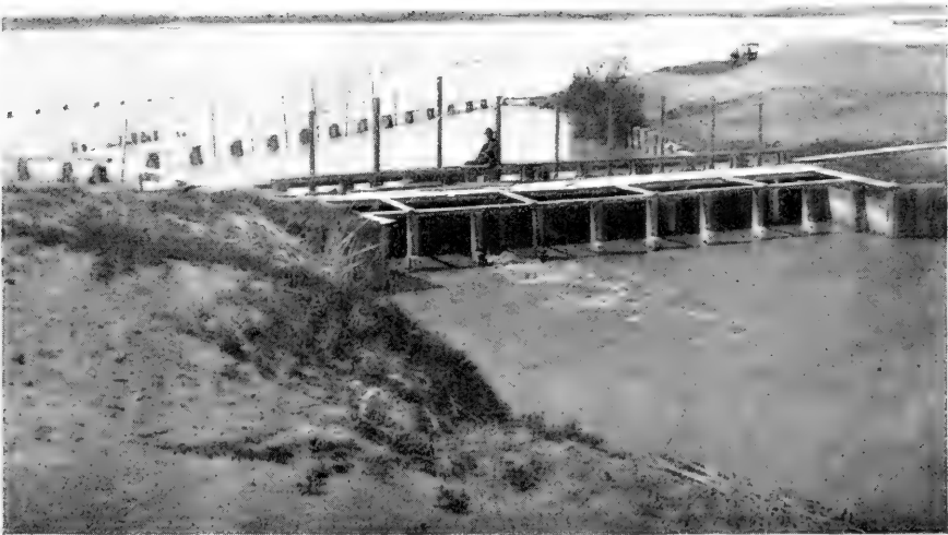
A Typical Headgate on the North Platte. There are 9 Gates, as Shown by Uprights
