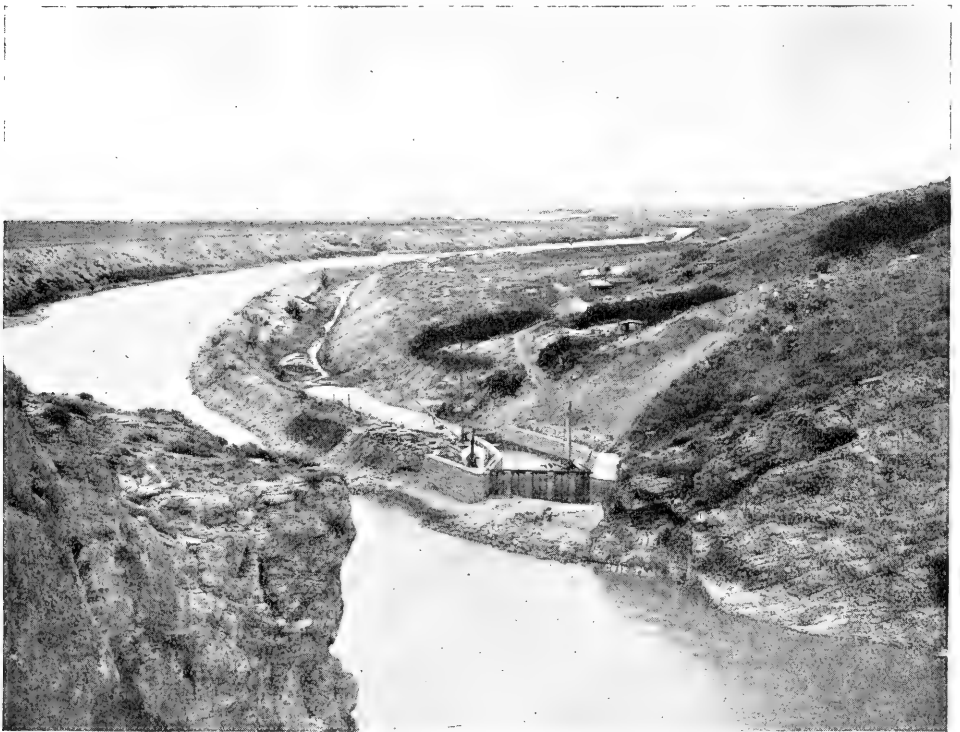
Headgates and Part of Canal, Bigham River
