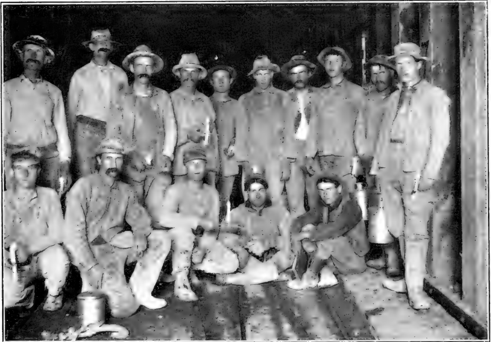
Workers in Gunnison Tunnel
