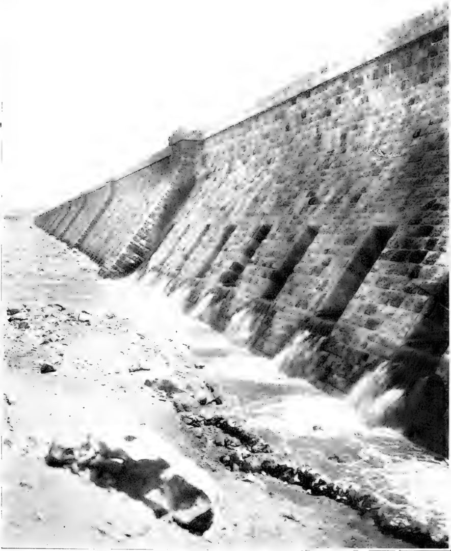
Water Flowing Through the Upper Tier of Sluices, Down-stream Side
