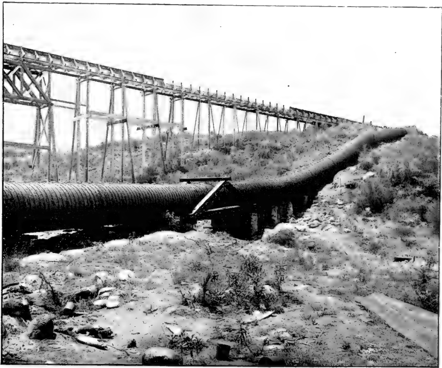
Conveyance of Water for Irrigation in Stave Pipes. Old Flume and New Redwood Stave Pipe Replacing It, Redlands Canal, California
