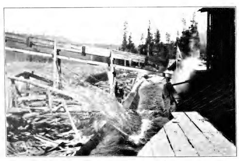
No. 6. THE SPLASH FROM A RAILROAD TIE THAT HAS JUST BEEN THROWN OFF THE CARRIAGE OF THE SMALL SAWMILL, INTO THE FLUME.
