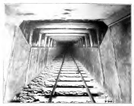
PLATE III. STEEL GAUGEWAY SUPPORTS IN ENTRANCE TO ALLPORT MINE. ALL STEEL AND CONCRETE
