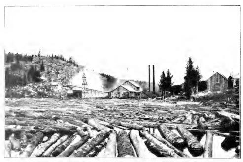
No. 5. THE LOG POND OF A SMALL SAWMILL LOCATED WITHIN THE BOUNDARIES OF THE FOREST. TIES, SMALL LOGS AND LARGE SLABBED LOGS ARE FLUMED TO THE LARGER MILL IN THE VALLEY.
