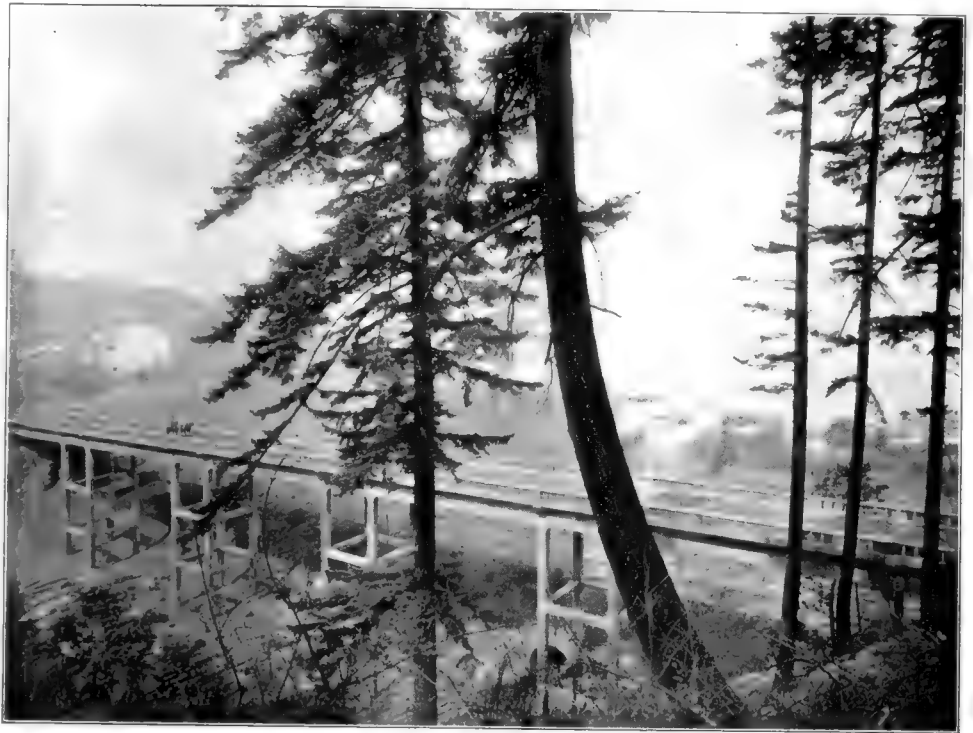
MCCORD CREEK BRIDGE
