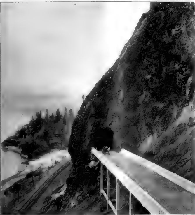
THE APPROACH TO A TUNNEL
