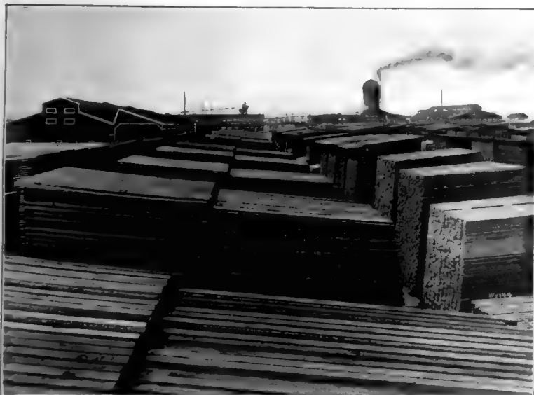
A LARGE AIR-DRYING YARD OF DOUGLAS FIR
