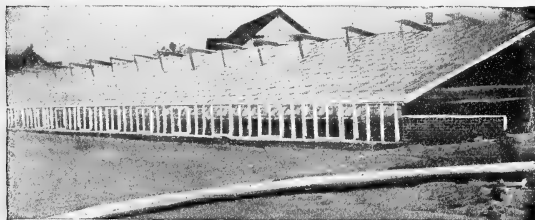
THE SOUTH ELEVATION, AND THE VENTILATORS.
