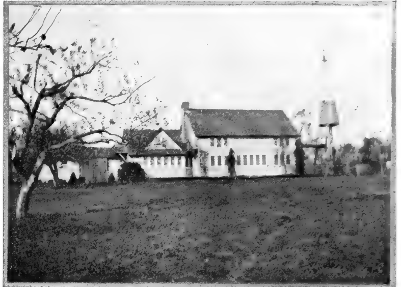
The house after the transformation
