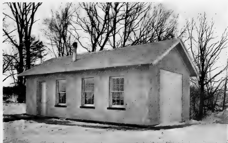
A garage and power plant can be combined, and such an equipment installed as that shown in the illustration to the right
