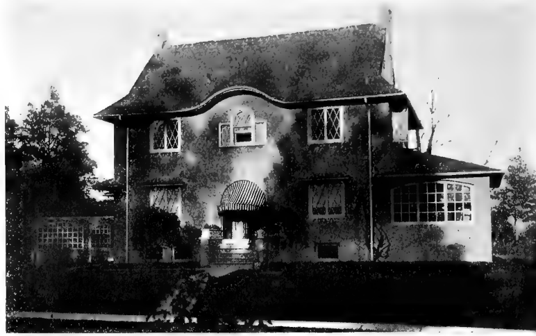
Floor plans and exterior of the stucco house owned by Mr. Pickslay. Oakley Manor, Mount Vernon, New York
