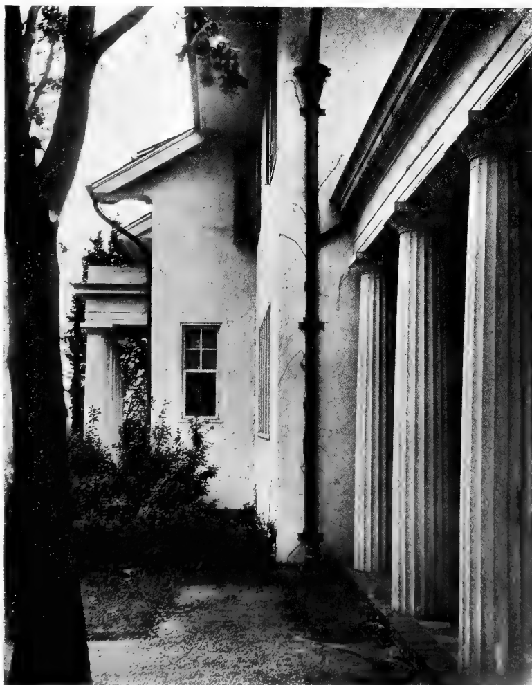
Detail of the pillars of the spacious piazza at the north end of the house
