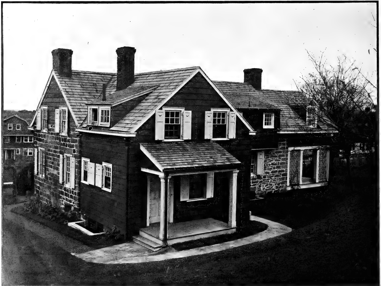
In order to meet the space requirements of the owners, a frame extension was added to the rear of the original structure and also the upper story wing shown in the right of the above illustration
