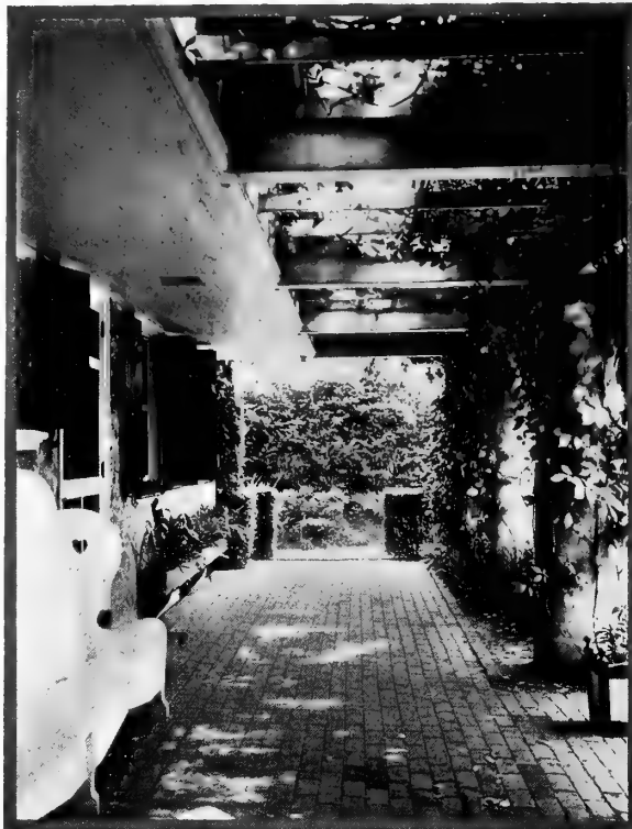
The brick-paved porch, whose floor is on a level with the lawn, instead of having a solid roof has staunch rafters spanning the space between the thick white pillars and the overhang
