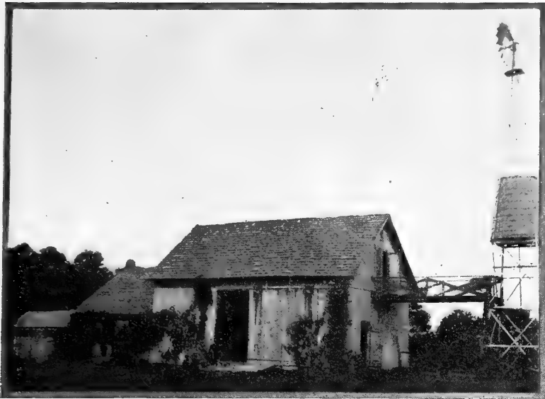
The old barn before remodeling
