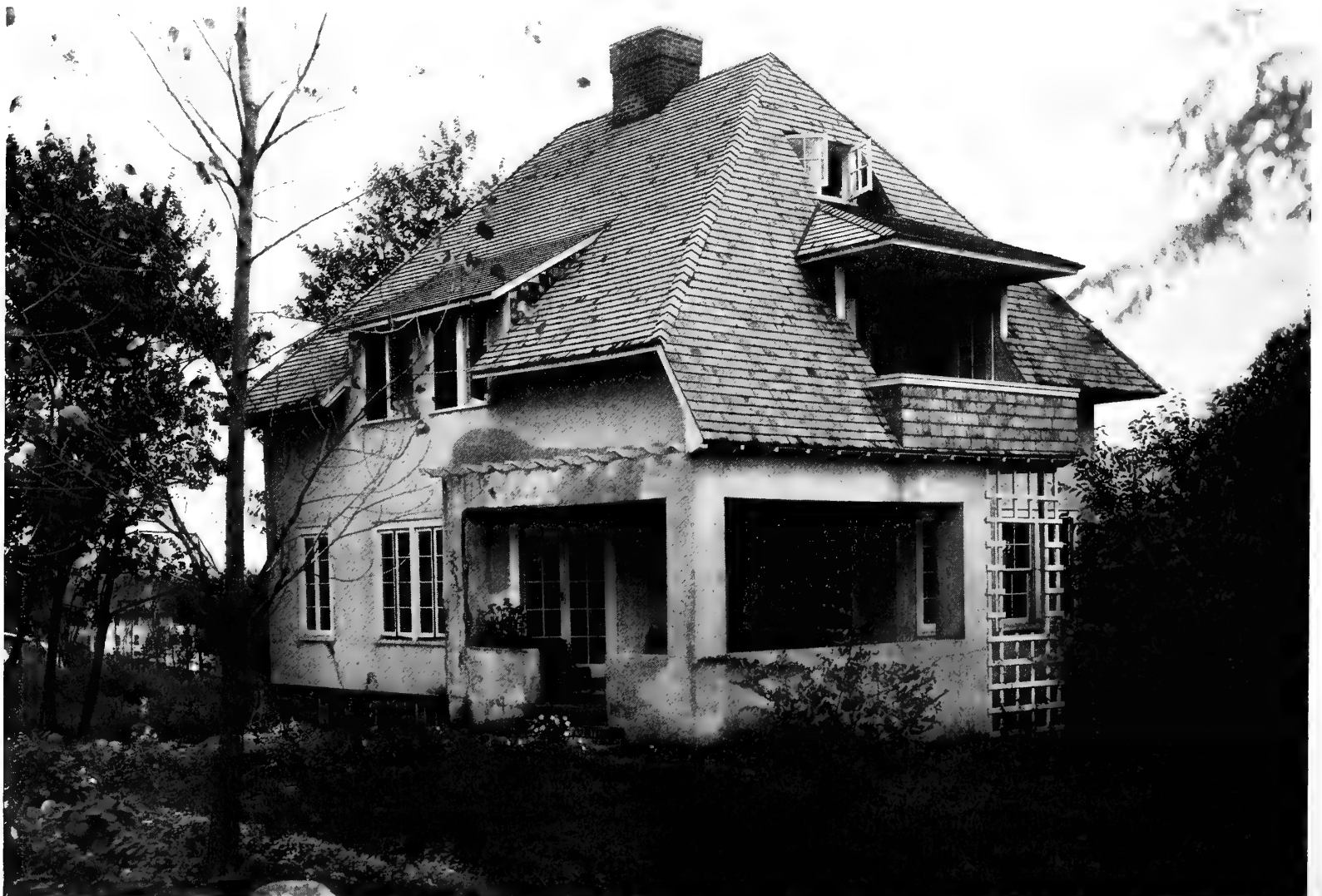
The home of Mrs. E. B. Winans, at Tuckahoe, New York, a very successful and attractive example of the small house of stucco
