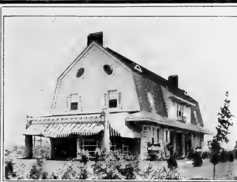
Stained with Cabot's Shingle Stains Aymar Embury II, Architect, New York
