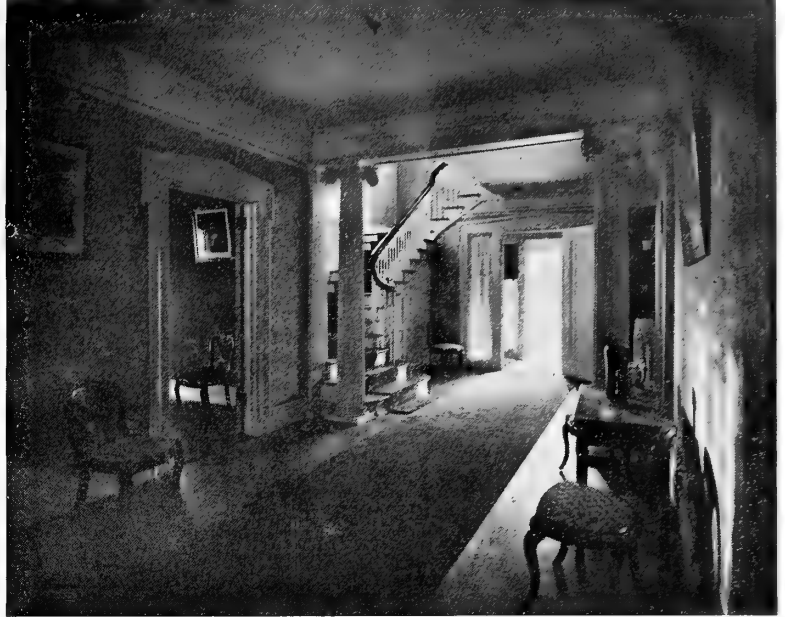
Hall, looking toward the entrance doorway
