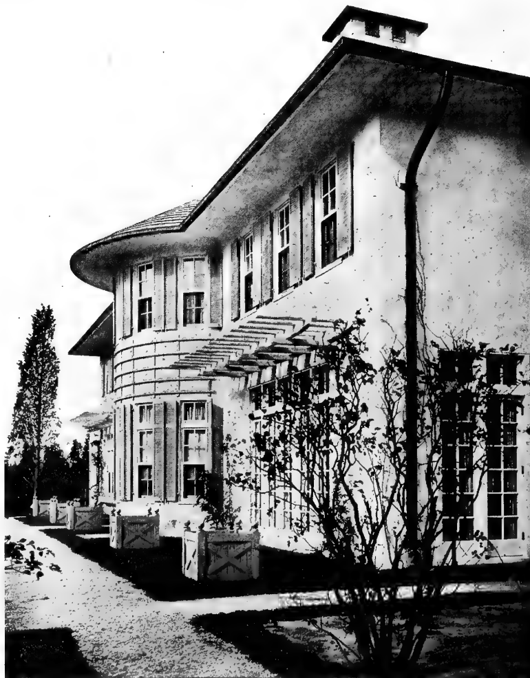
The plastered soffits and two-story circular bay form particular features of this interesting Long Island house
