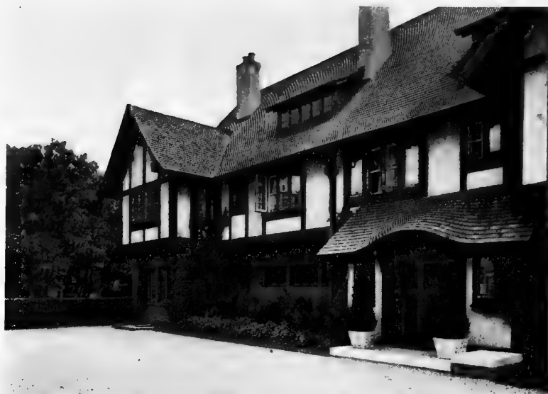
The entrance doorway
