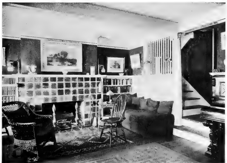
The living-room of the Clark house showing stairway
