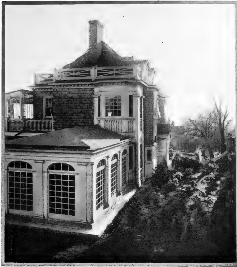
The Callaway house as seen from the roadway
