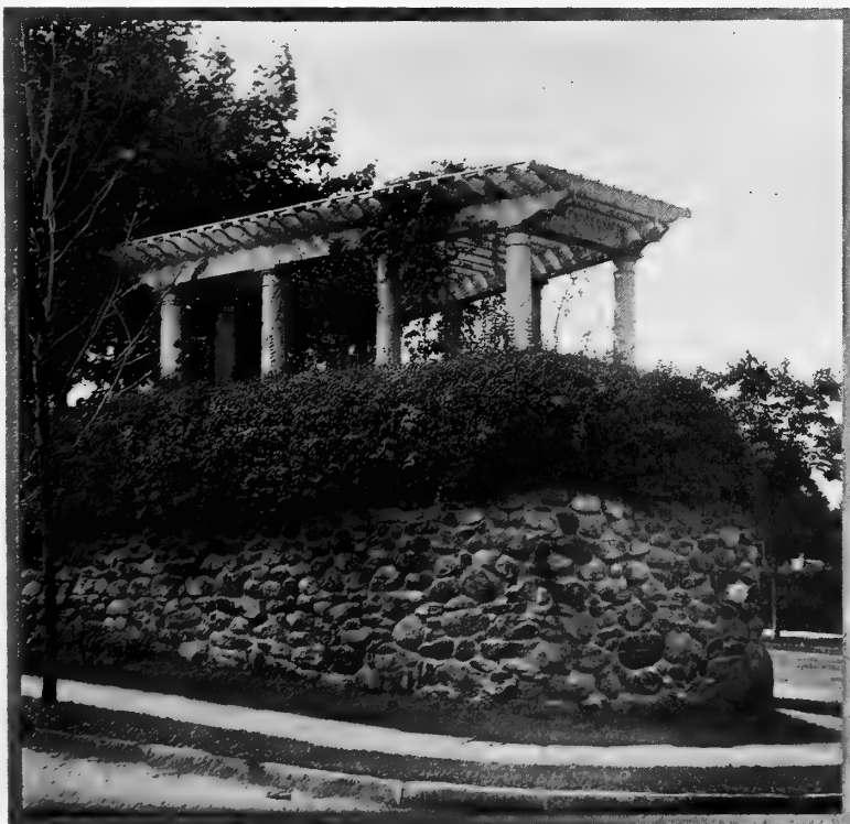
The sloping triangular corner here shown was walled and brought to a level with the lawn back of it, a pergola being added, furnishing a delightful outlook.
