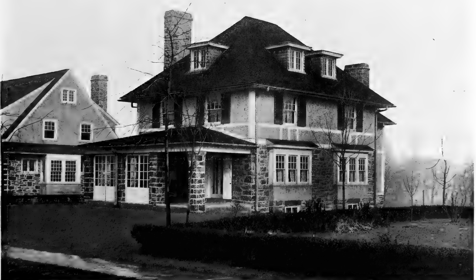
The total cost of this particularly attractive stone and stucco house when completed was kept well within $6,700
