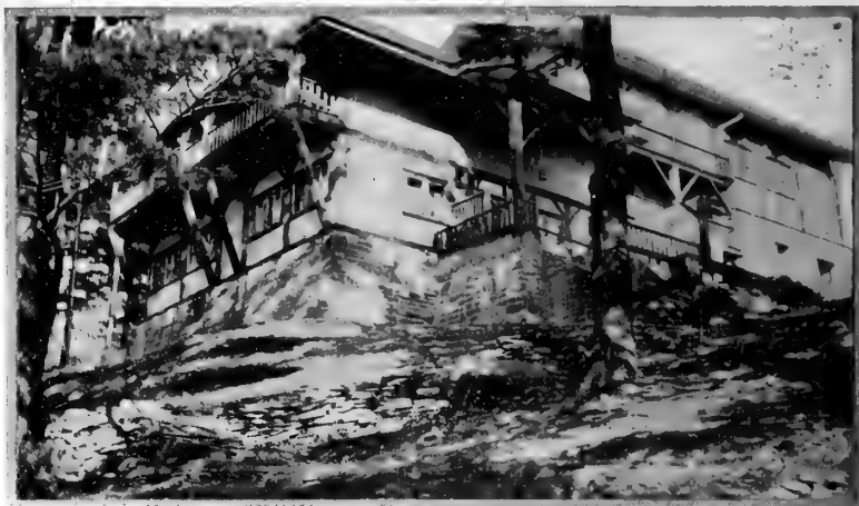
View of the house showing long upper balcony
