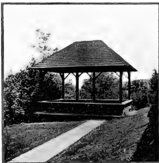
A house to shelter the sand pile
