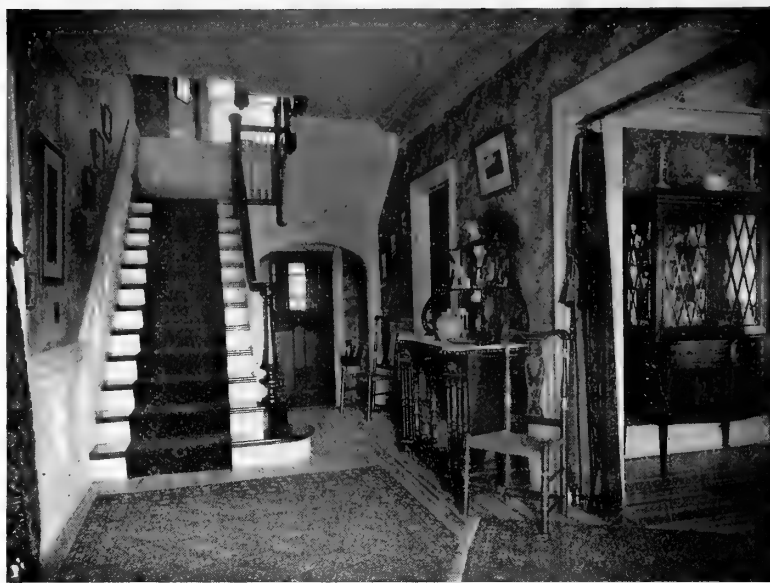
The hall and stairway with its wainscoting and graceful baluster and newel
