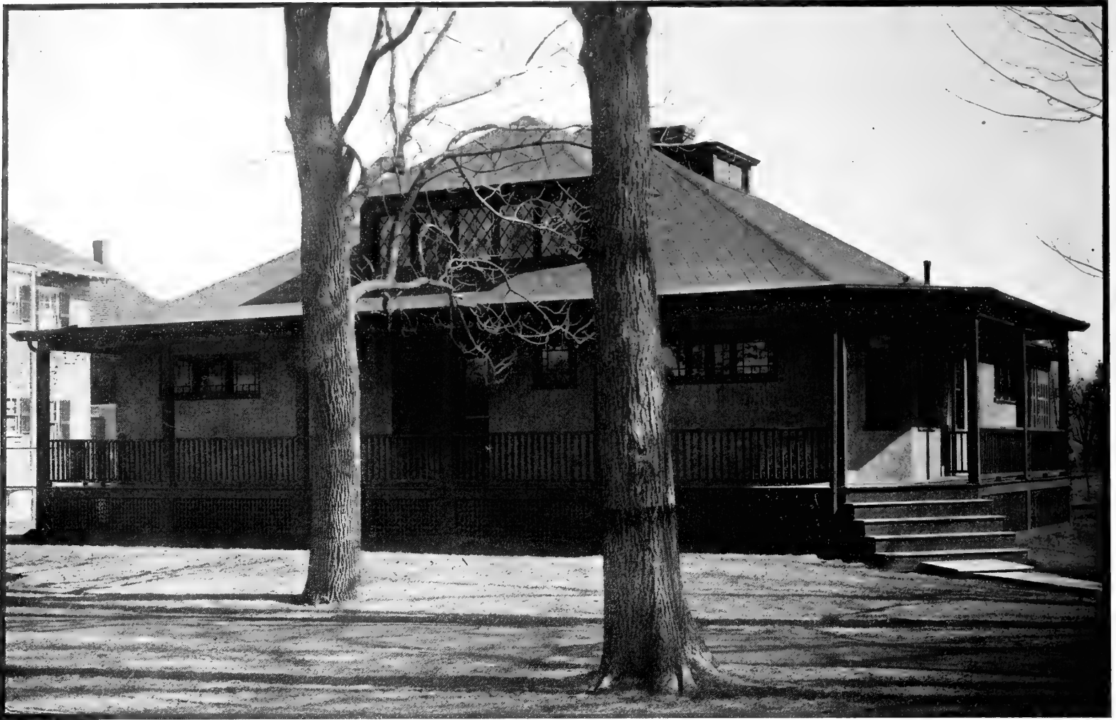
This unconventional bungalow is built of terra cotta hollow tile, covered with rough plaster, and was designed by its owners
