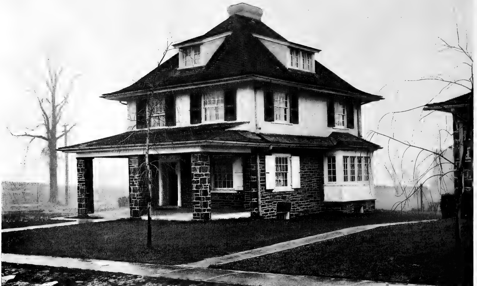
Here one sees a small house of stone and stucco, a paragon of neatness and attractiveness, costing but $5,500
