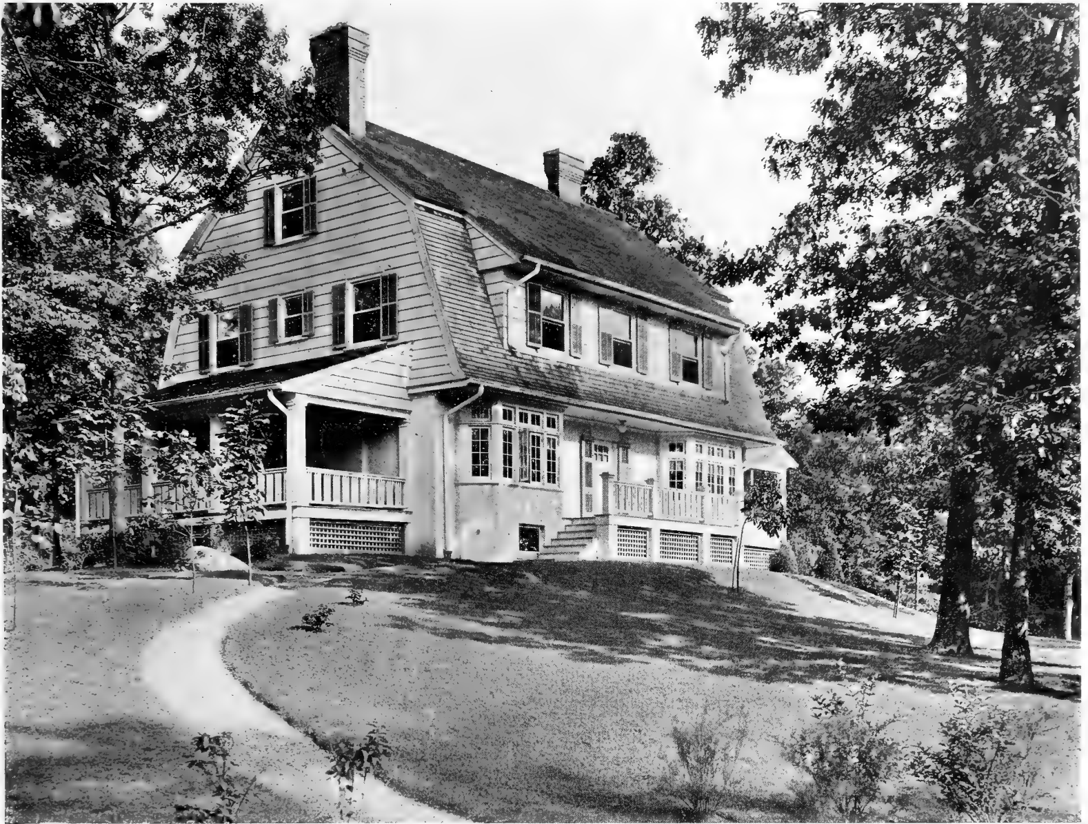
The home of Dr. Dwight E. Marvin, at Summit, New Jersey, is an unusually successful example of the gambrel roof type of house
