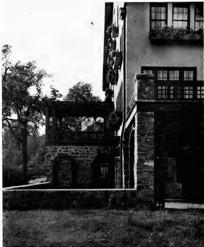
The pergola is set upon the high stone walls of the old structure
