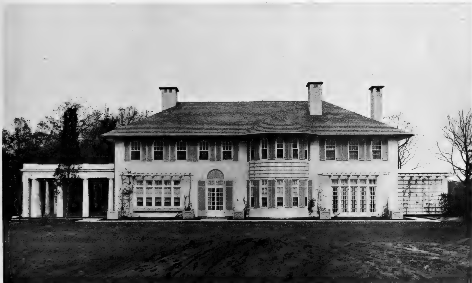
This view shows the façade fronting the uncompleted lawn, and it presents a remarkably fine example of unusually successful fenestration
