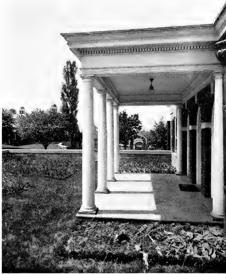
One view of the entrance portico
