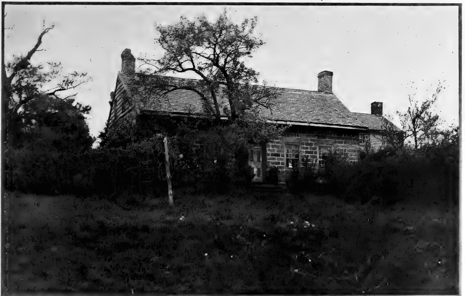
This picturesque old stone farmhouse required very little external remodeling to make its interior light and roomy
