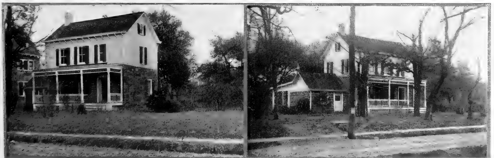
The old house as it stood when purchased before it was burnt. The superstructure had evidently been added to the original stone wall
