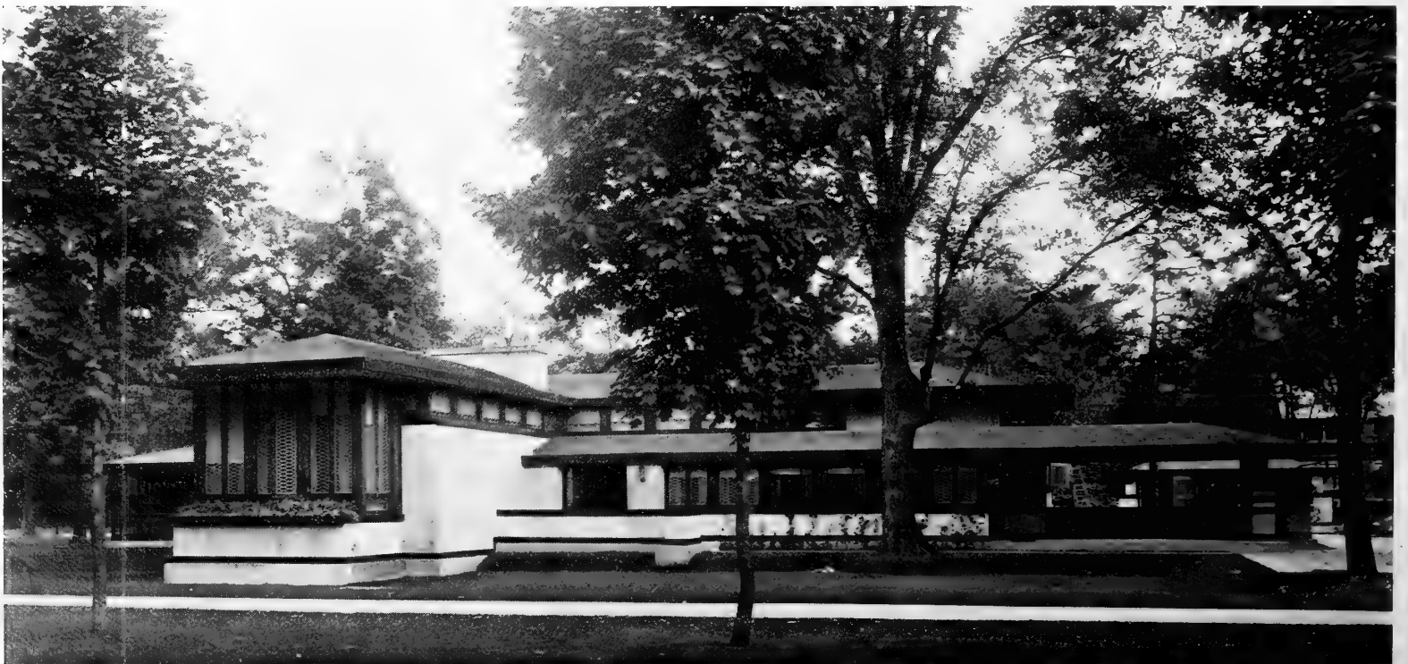
A residence in the "Western" style of architecture, at Wilmette, Illinois, one of Chicago's most attractive suburbs
