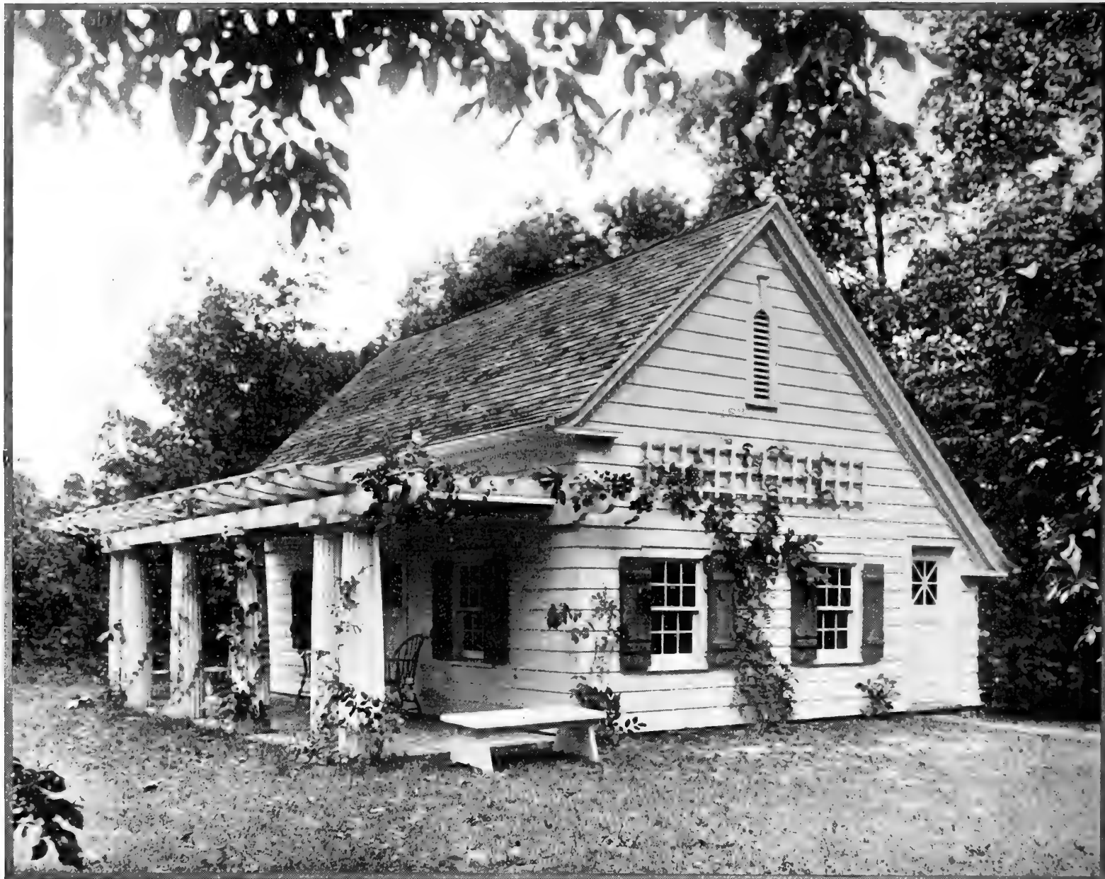
A playhouse upon a large country estate where it agrees in style with the other buildings
