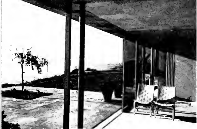
Above and below, walls of heat-resistant glass roll open to join living room with terrace, ocean view.
