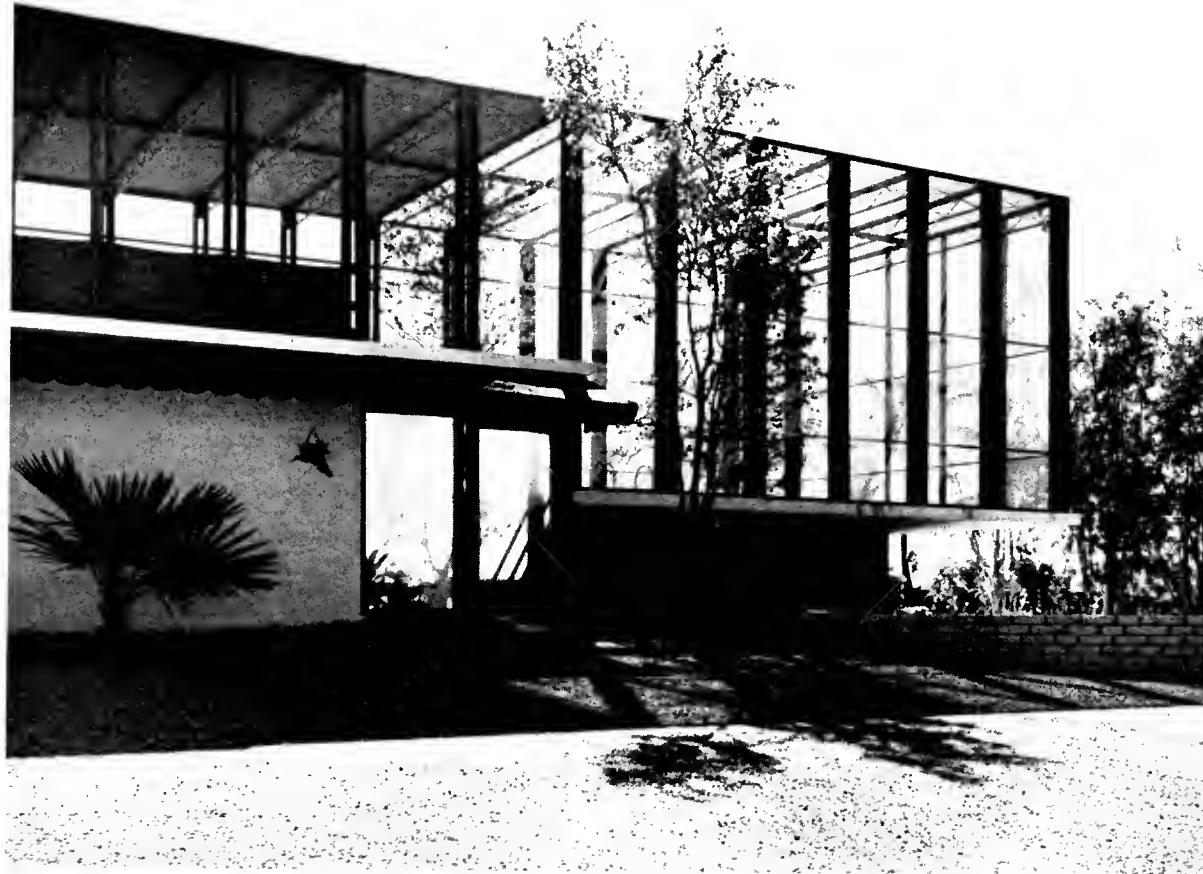
Above: the entrance side with swimming pool at right.
