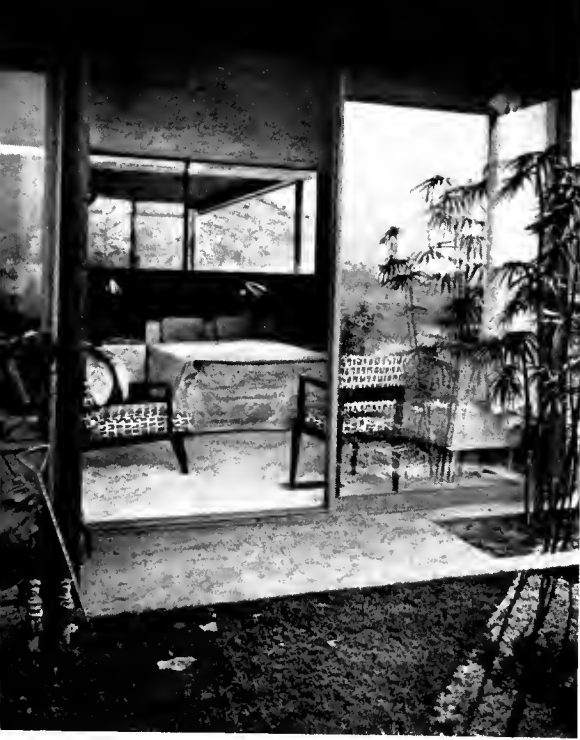
Above, a view into the smaller bedroom. The sliding glass walls are placed back of the outer line of the concrete-floored, steel-roofed structural grid, with the pipe columns exposed.
