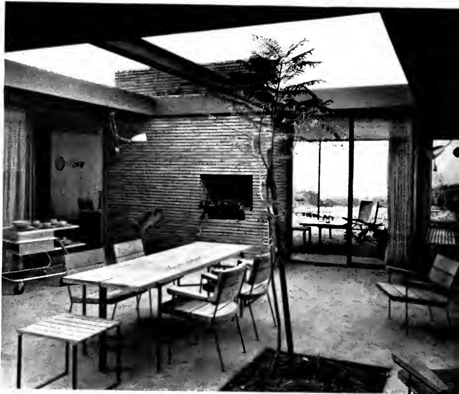
Above, a view into the smaller bedroom. The sliding glass walls are placed back of the outer line of the concrete-floored, steel-roofed structural grid, with the pipe columns exposed.
