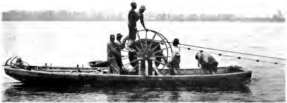
The crew walk up the spokes of the wheels as on a ladder thus causing the reel to revolve and wind up the seine
