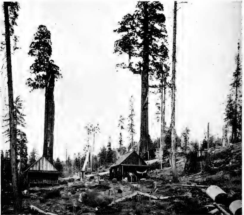
Typical appearance of land near a sawmill where the bigtree forest has been cut. None of the government's bigtrees are being cut at present
