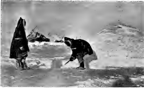
Keystone of dome of snow house about to be put in place
