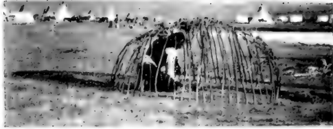
Building the frame of willows
