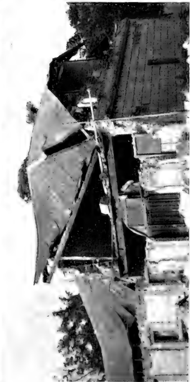
The British Legation after the shocks of December 25 and 29, and from the same point of view after the shock of January 3. Note the complete collapse of the second story in the later photograph. This last shock finished the work of destruction. What the others had spared, it shook down.
