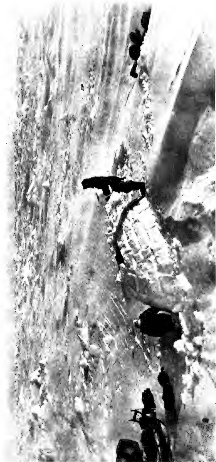
In the construction of a snow house about forty-two blocks, 24 x 18 x 4 inches in size, are used. When traveling over sea ice, we made a new house each night, consuming in time about fifty minutes
