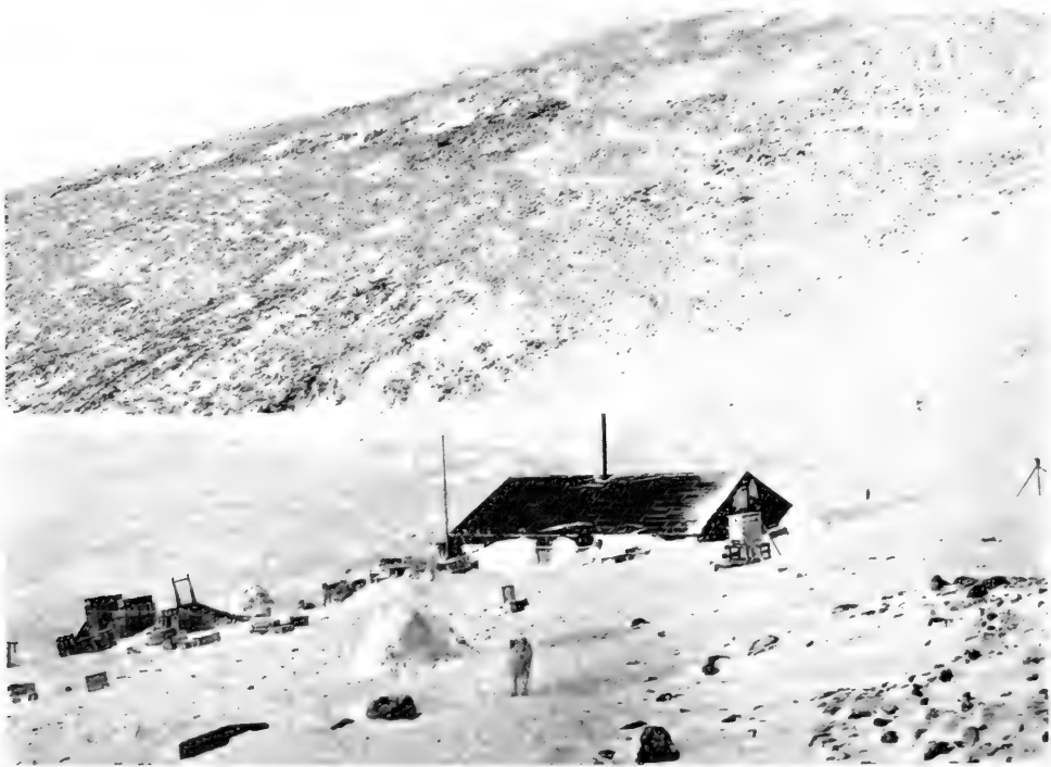
This is Borup Lodge, headquarters of the Crocker Land Expedition at Etah, North Greenland, as seen in early spring from the hill above. The house is one of the warmest buildings ever constructed in the North, the walls being double with a four-inch air space. It contains a large living room, four sleeping rooms, a work room, an electrical room, and a photographic dark room.
