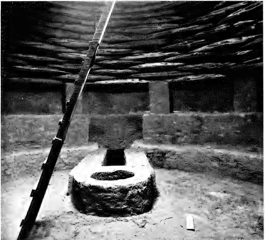
A kiva with reconstructed roof.—The entrance is through a hatchway in the center of the roof (see view above ground on page 602). The excellent architectural principle involved in the construction of this type of covering for a circular chamber is one of the highest tributes to the mechanical skill of the ancient Pueblos. Pillars of masonry support the roof, which is a cribbing of timbers in the form of a truncated cone. With its flat top and sloping sides, this sort of roof has the strength and permanence of a dome, and the neatly dressed timbers placed in regular rows impart beauty and dignity to the chamber which they enclose
