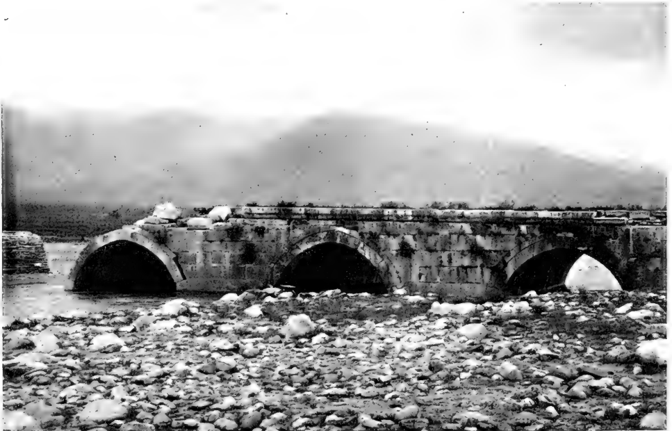
Marble bridge at the Ming tombs.—The bridge has been broken away at the end and within a few years will be entirely destroyed unless some action is taken to preserve it
