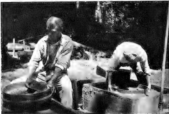
Two steps in the process of separating the diamonds from the gravel.—The man at the right is swirling some gravel in his sieve to send the diamonds to the bottom. The other man is scooping out of his sieve the top layer of residue gravel from which the diamonds have been jiggled to the lower layer. A careful jigger rarely loses a diamond from the mass of gravel
