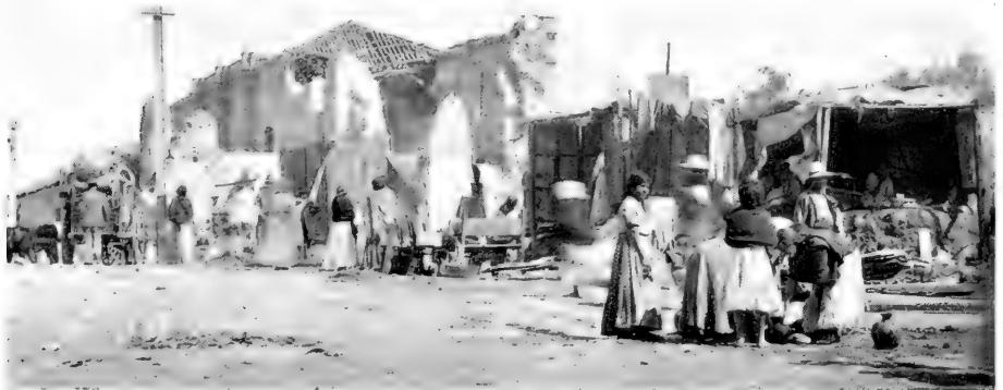
Church of the Sanctuary.—In the foreground are temporary shelters with sides of matting and cloth and roofs of sheet iron
