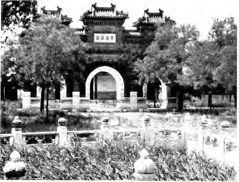
Pai-lou in the courtyard of the Hall of Classics. — An atmosphere of neglect, decay, and dilapidation rests on the temple, creating in all observers a feeling of sadness that so much beauty is left to perish.
