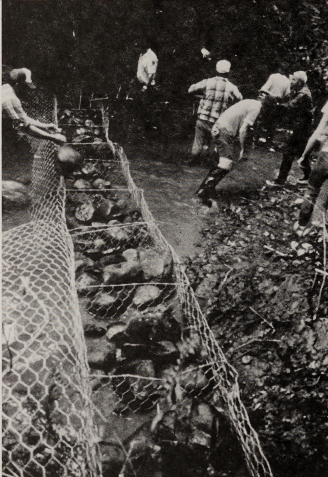
5. Volunteers fill wire gabion baskets with rocks used to create pool and spawning habitats and protect streambanks.
