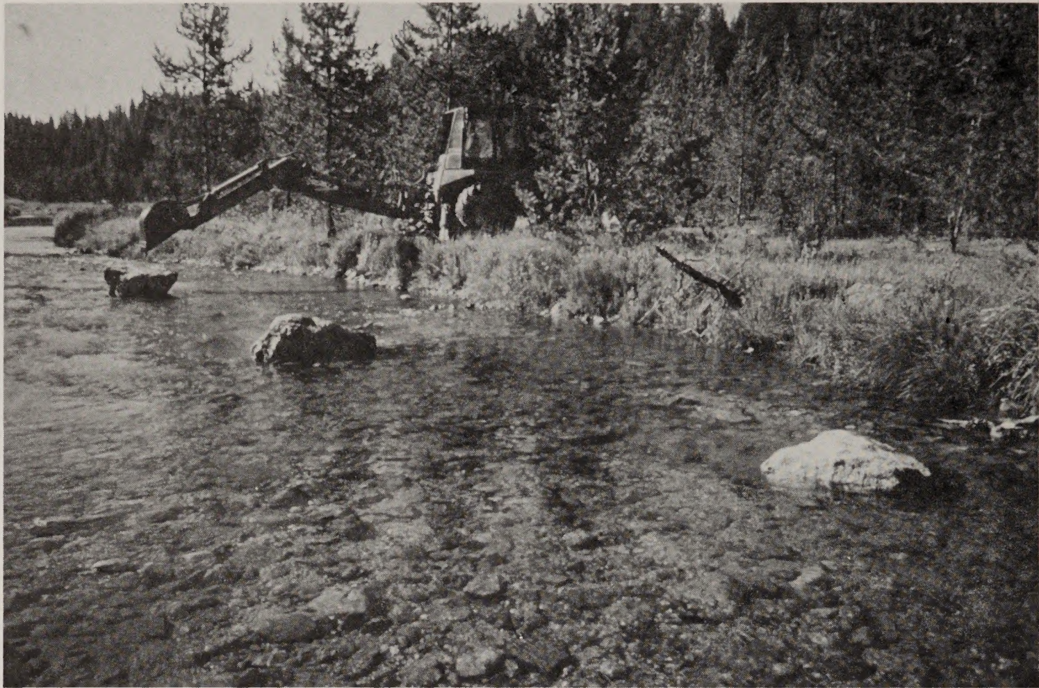
12. Large boulders are individually placed by heavy equipment to create pool habitats of young and adult fish.
