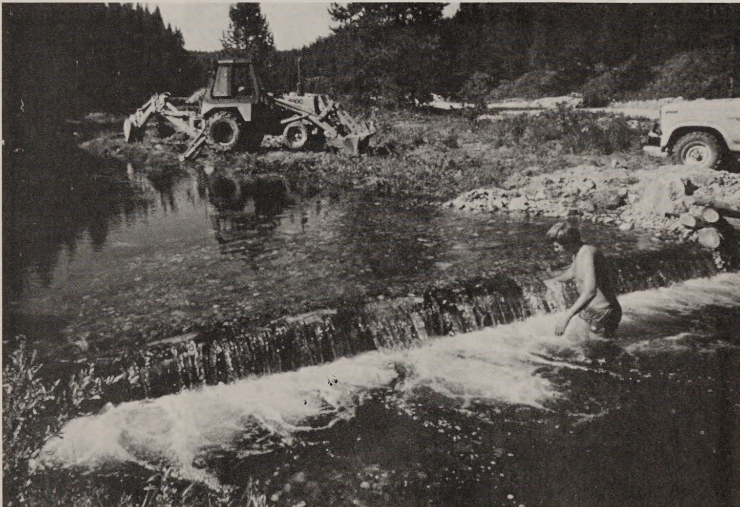
4. Completed "K" dam creates a spawning area above and excellent pool habitat below the dam.
