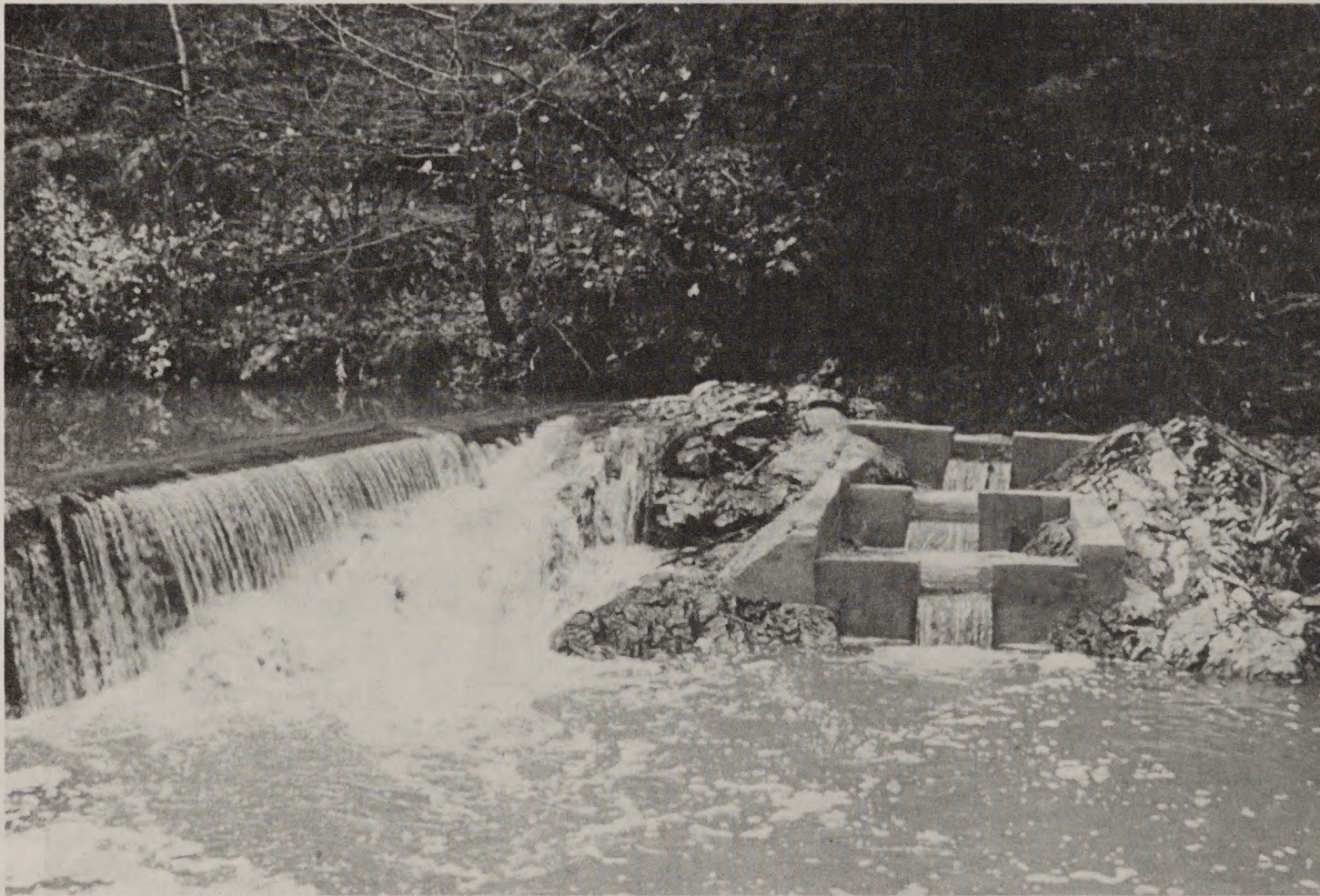
9. This concrete step-and-pool fishway was constructed at a low irrigation dam to provide anadromous fish easy access to upstream spawning areas at all streamflows.
