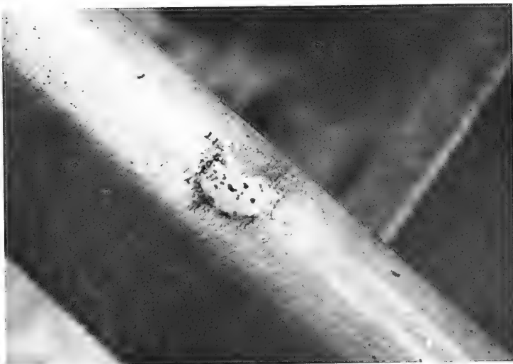
Figure 13. Same area as in Figure II with rust staining removed.
