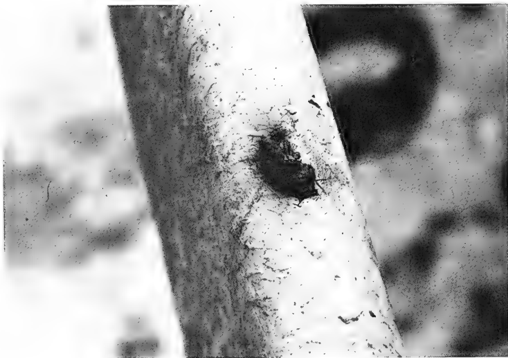
Figure 11. Rusted area of middle frequency antenna.
