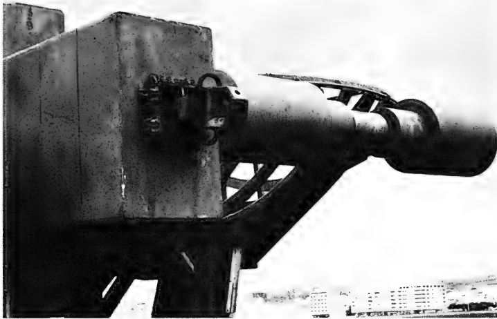
Figure 16. Main lifting eye at top of foam tower.
