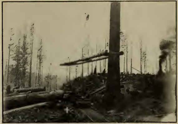
FIG. 4C—10"x12" LOADER WITH MCLEAN BOOM
