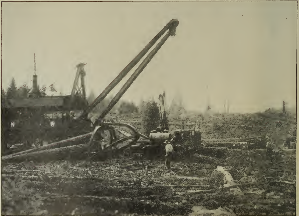
FIG. 6—MCGIFFERT LOADER ("JAMMER") AND TRACTOR ARCH UNIT AT LANDING
