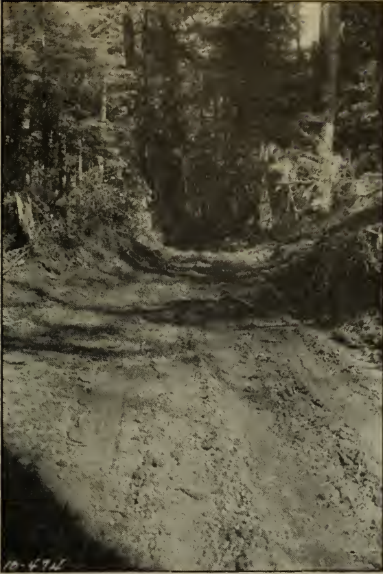
FIG. 46—(LEFT) TRACTOR ROAD CONSTRUCTED WITH "BULL-DOZER" AT A COST OF $200 A MILE; (UPPER RIGHT) HAULING A 5.6 M FT.B.M. LOG 1,100 FEET TO THE LANDING AT A COST OF 22 CENTS PER M; (LOWER RIGHT) ROADING A 6.2 M FT.B.M. LOG WITH THE AID OF A HELPER TRACTOR 48 HOURS AFTER A HEAVY RAIN
