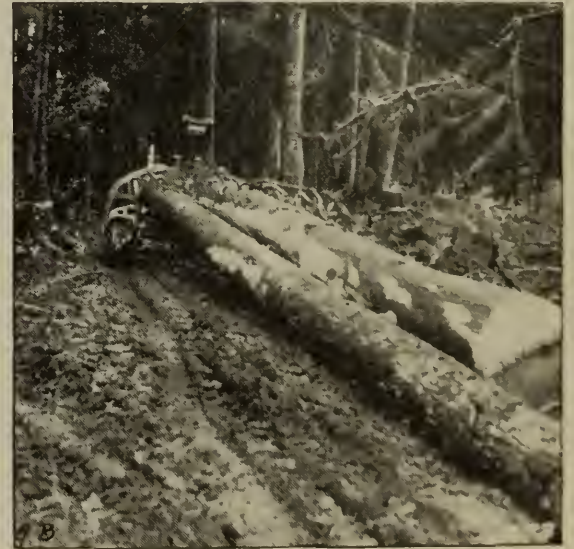
FIG. 47—(LEFT) WINDING TRACTOR ROAD ON 20 PER CENT GRADE; (RIGHT) BUTT LOGS FROM TREES UNDER FIVE FEET IN DIAMETER WERE USUALLY TAKEN IN 56 OR 64 FOOT LENGTHS
