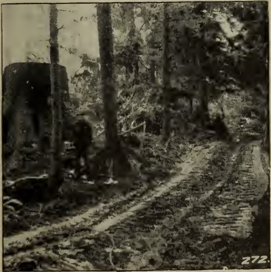
FIG. 47—(LEFT) WINDING TRACTOR ROAD ON 20 PER CENT GRADE; (RIGHT) BUTT LOGS FROM TREES UNDER FIVE FEET IN DIAMETER WERE USUALLY TAKEN IN 56 OR 64 FOOT LENGTHS
