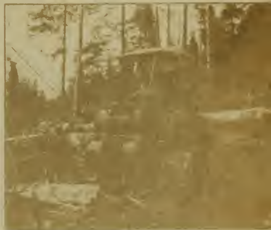
FIG. 4. TRACTOR DONKEY USED FOR HIGH LEAD YARDING.
