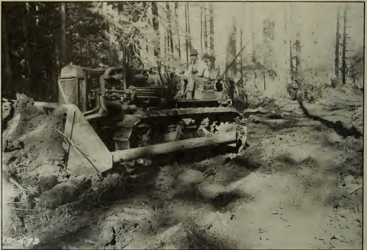
FIG. 45—THE "BULL-DOZER" AT WORK. GRADING IS PERFORMED MOST EFFICIENTLY BY WORKING DOWNHILL
