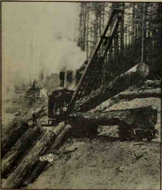
FIG. 4B—LOCOMOTIVE CRANE WITH HEEL BOOM
