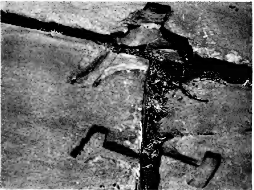
FIG. 38. Typical wall construction and detail of sockets for cast copper cramps or tie bolts in stone paving at Tiahuanaco.
