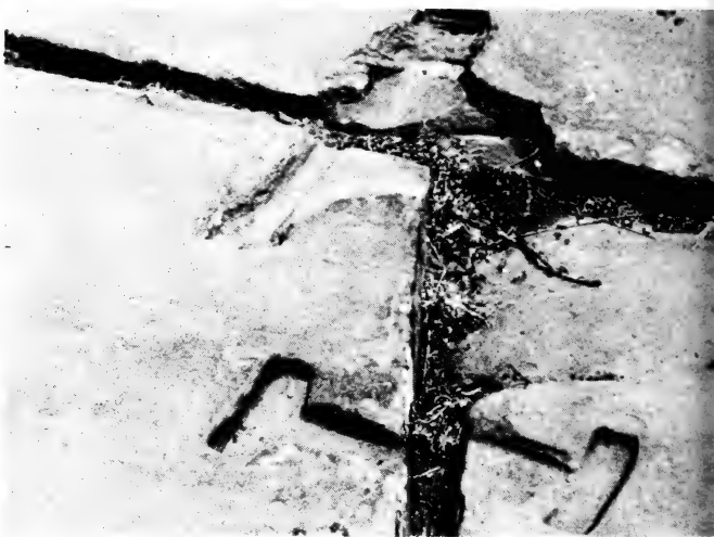
[20] Typical wall construction and detail of sockets for cast copper cramps or tie bolts in stone paving at Tiahuanaco.
