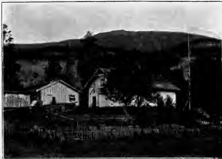
THE FORSTASSISTENT'S HOUSE.
