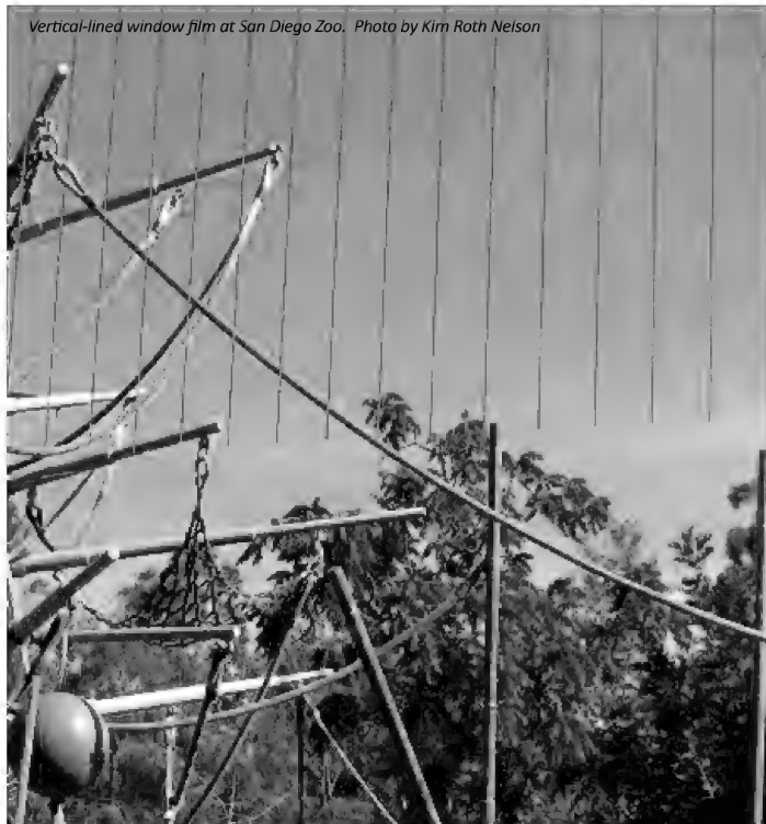
Vertical-lined window film at San Diego Zoo. Photo by Kim Roth Nelson
